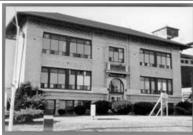
Ford City School, 1917 3177 Riverside Dr. E. (Demolished)
