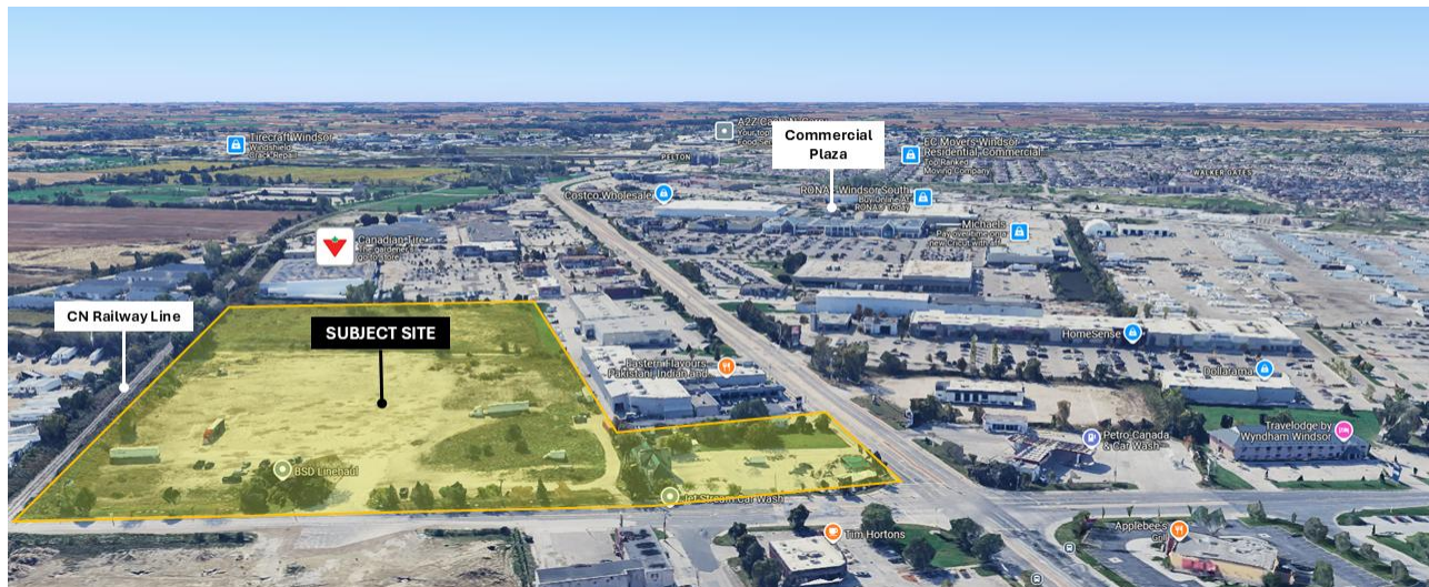
Figure 5 – View of the Subject Site facing South
