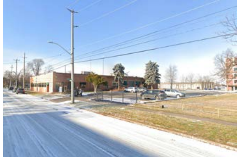
Figure 1.4 - Site looking west from Assumption St
