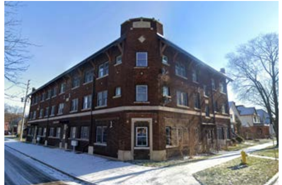
Figure 1.10 - Low-rise apartment along Assumption St
