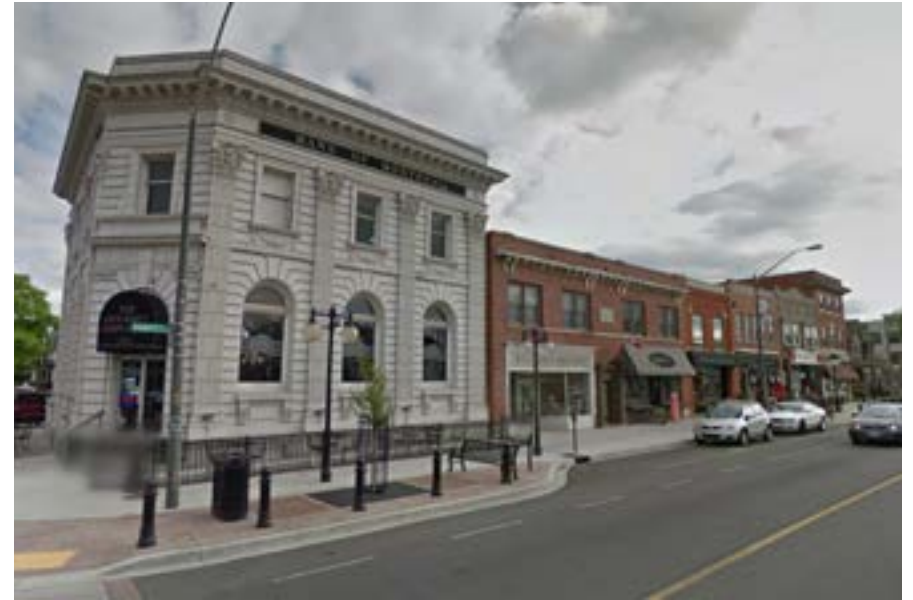
Figure 1.9 - Main street corridor along Wyandotte St E
