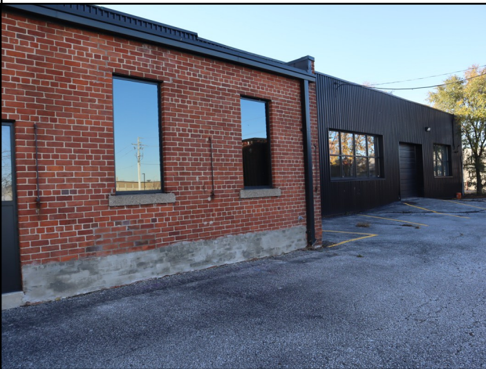
Photograph 3: View of the site building facing southwest.
