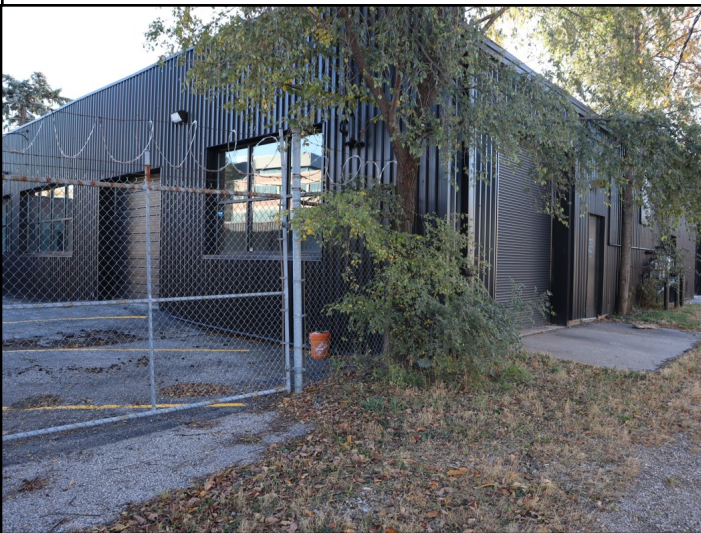
Photograph 7: View of the northwest corner of the site building. Image taken from the west adjacent alleyway.
