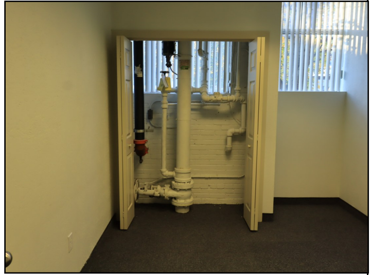
Photograph 14: View of a vacant room and piping observed in a closet of Unit #200.
