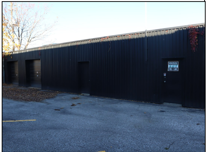
Photograph 4: View of the storage building located in the northwest corner of the site.
