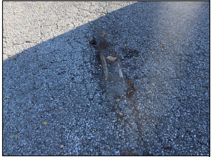
Photograph 6: Exposed portion of a railway spur located in the north portion of site within the asphalt parking lot.
