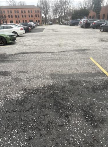
IMAGE 5 ASPHALT PARKING LOT
