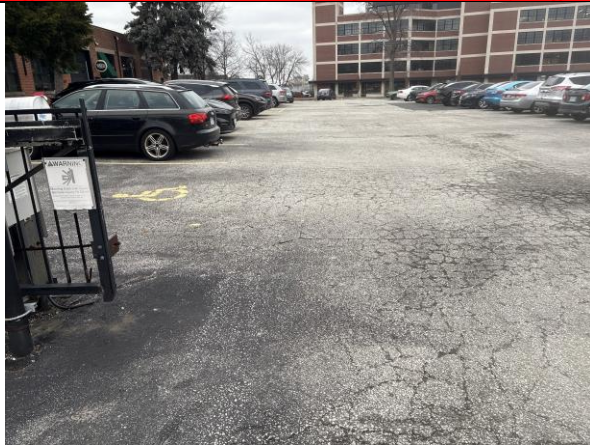
IMAGE 7 ASPHALT PARKING LOT
