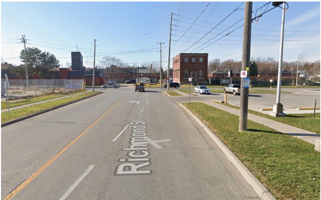
Figure 6: Looking West on Richmond Street toward Walker Road
