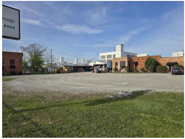
Image 8: Subject property, facing north to parking area and existing building.
