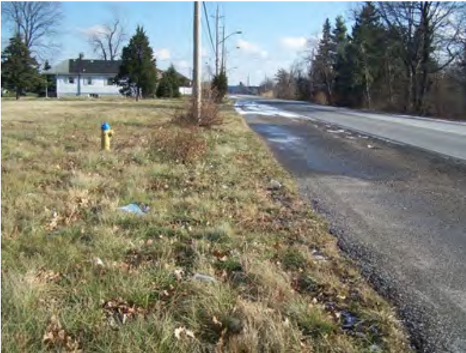
Plate 3: Looking east along North Talbot Road from the current 6th Concession Road intersection, showing the paved shoulder & water main but no ditching.
