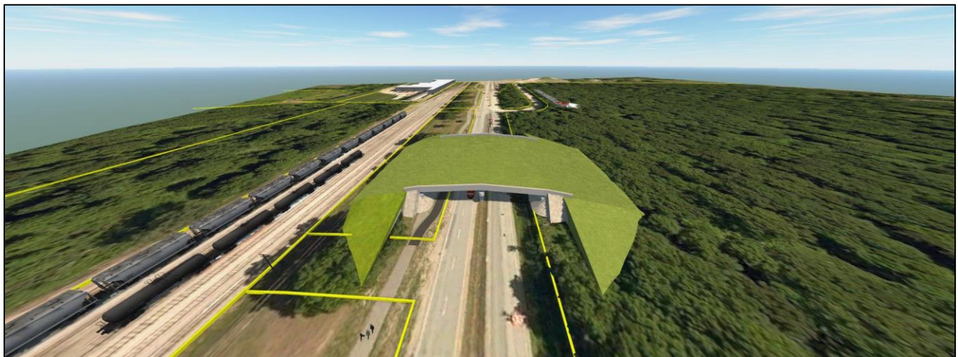
Figure 8-6: Initial Design Option 3 - Wildlife Overpass (2-Span Bridge) – Profile View
