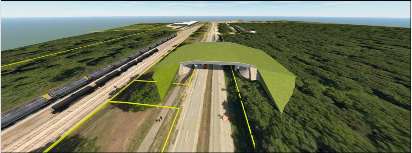
Figure 8-2: Initial Design Option 1 - Wildlife Overpass (3 Span-Bridge) – Profile View
