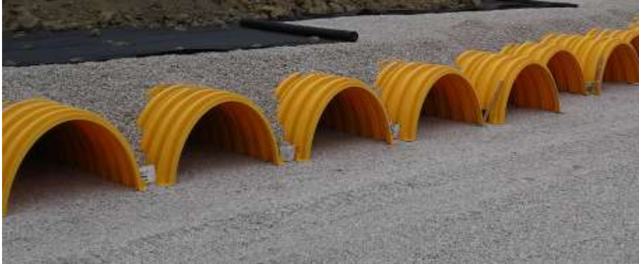
Underground Stormwater Detention System
