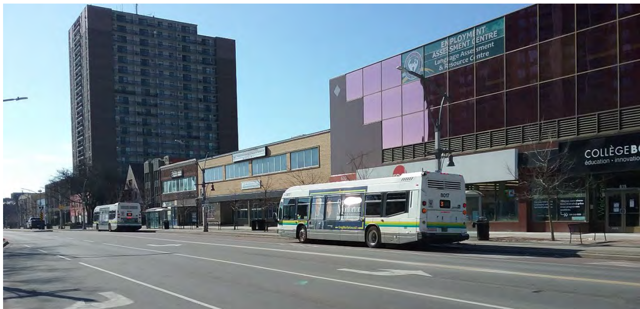
Figure 68 Transit Windsor On-Street Terminal at Ouellette and Wyandotte
