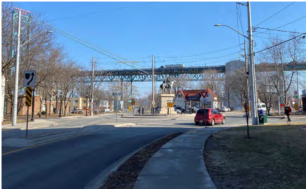
Figure 124 Example of a Roundabout Used by Transit Windsor
