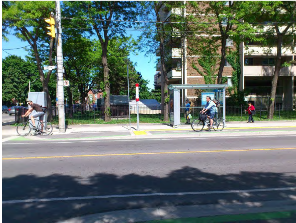
Figure 57 Example of a Shared Cycle Track Bus Stop
