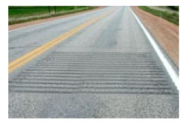
Figure 2: Transverse Rumble Strip Example (Source: Neal Hawkins/lowa DOT)
