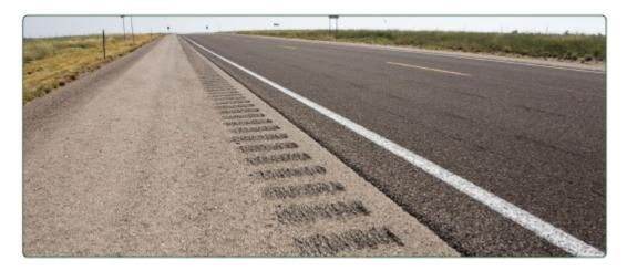
Figure 8: Pavement Edge Rumble Strip Example (Source: FHWA)
