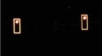
Figure 1: Retroreflective Backboards (source: Virginia DOT / FHWA)
