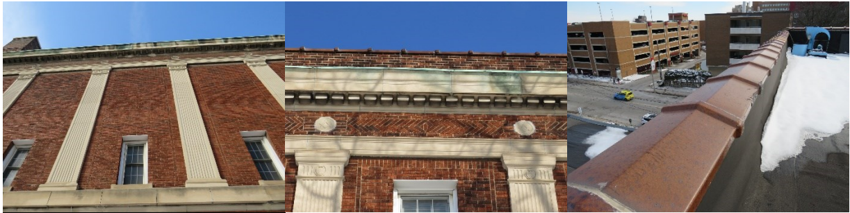
Photo of the side and front flashing and parapet, with the clay tile parapet coping on right.
