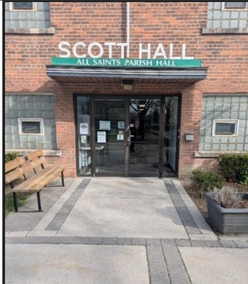
Photo 2 External View to South Entrance
