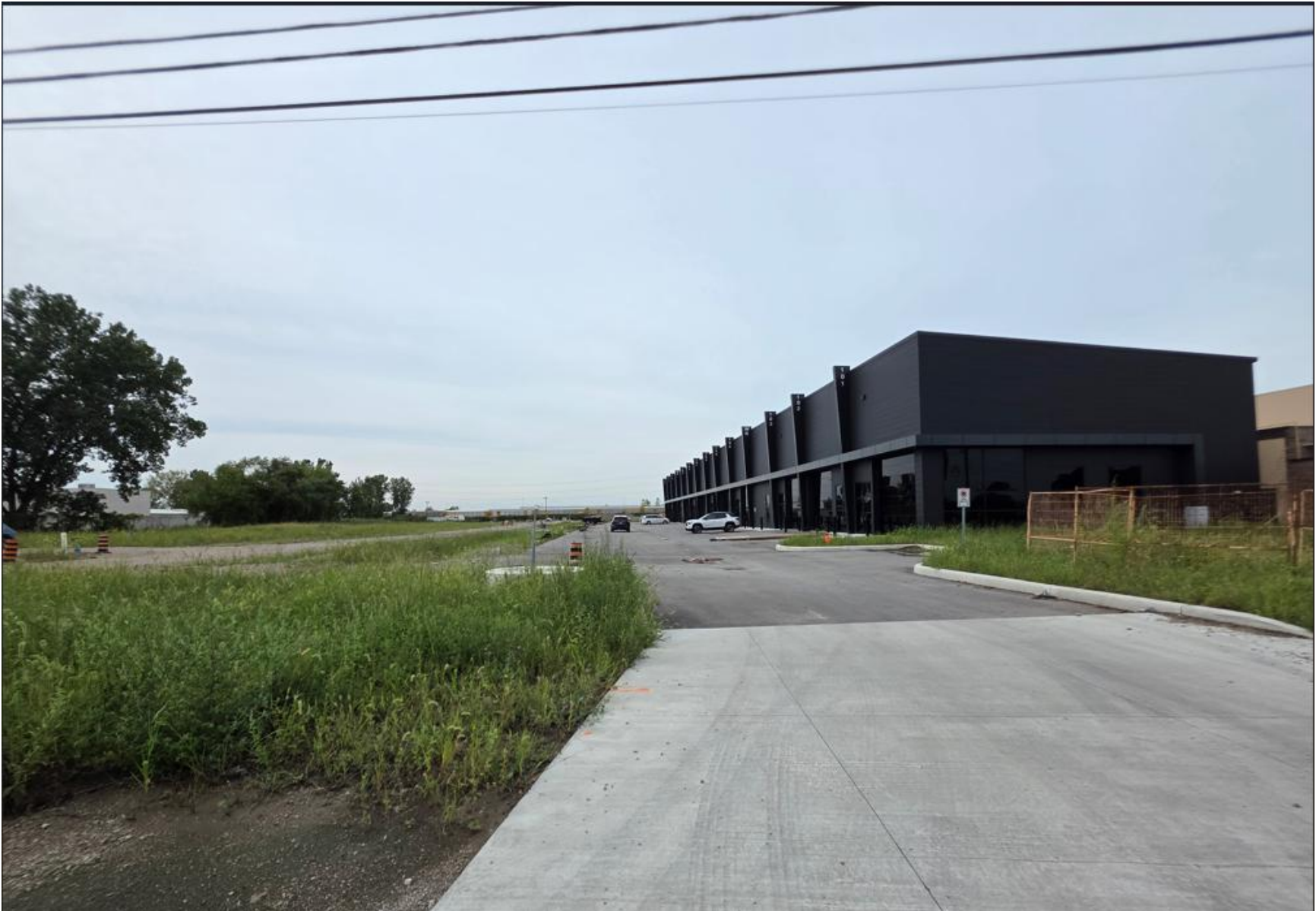
VIEW OF SUBJECT SITE FROM NORTH SERVICE ROAD EAST, SHOWING THE NEWLY CONSTRUCTED BUILDING 1
