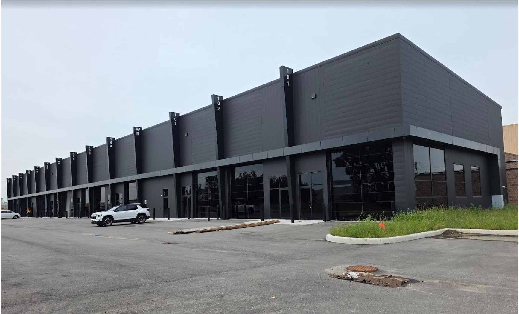
A CLOSE VIEW OF THE NEWLY CONSTRUCTED BUILDING 1
