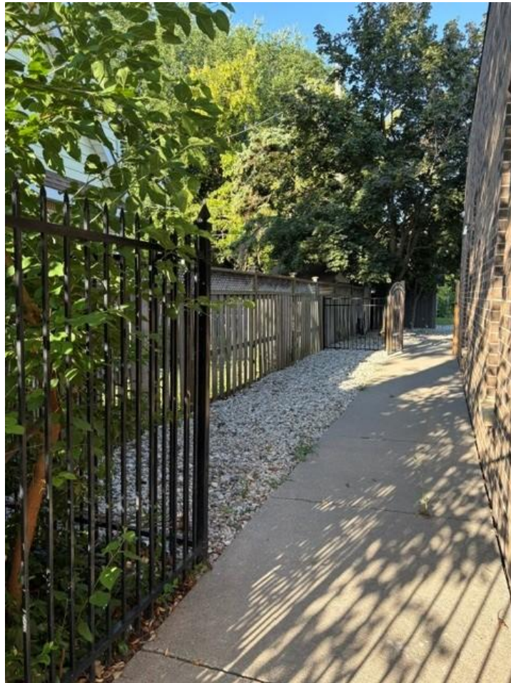
Figure 3 – View of wood fence encroaching on southerly edge of alley
