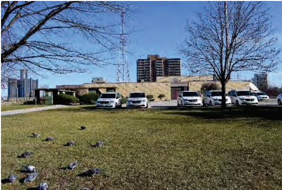
Photo 25: Front (west) façade, looking east
