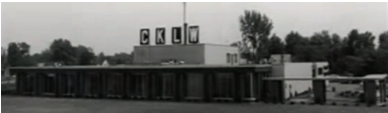
Plate 2 CKLW following completion of Hilliker’s addition (Kryger 2020)
