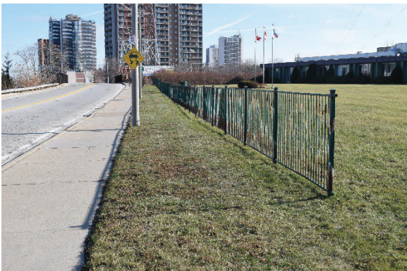
Photo 21: Metal fence, looking east
