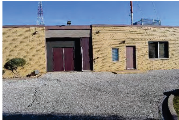
Photo 34: Secondary entrance and windows, looking east
