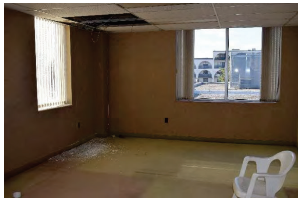
Photo 76: Representative second storey office, looking west
