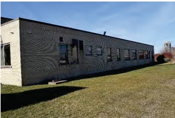
Photo 41: East façade, looking north
