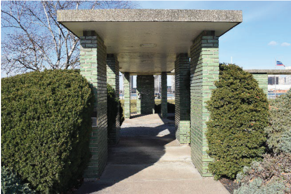
Photo 27: Breezeway south entrance, looking north
