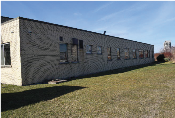
Photo 41: East façade, looking north
