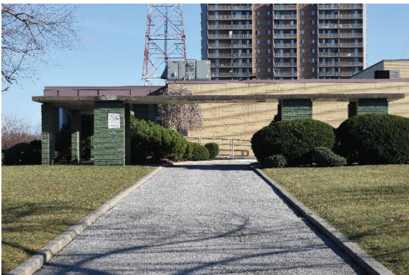
Photo 13: Driveway as it passes under breezeway, looking east
