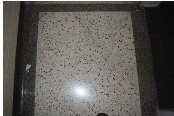
Photo 68: Terrazzo washroom flooring, representative photo
