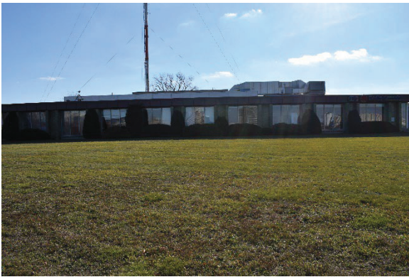
Photo 35: North façade, looking south
