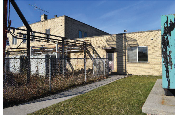
Photo 46: East side of south façade, looking north
