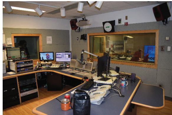
Photo 56: Studio B control room, looking north
