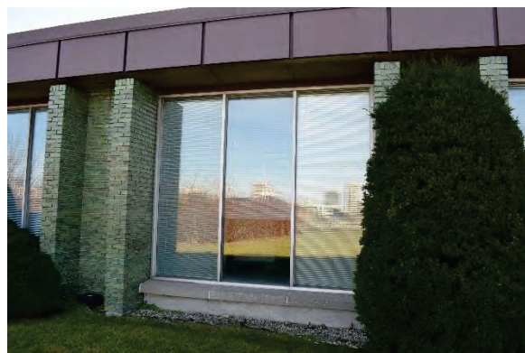
Photo 38: Window details and metal flashing, looking south
