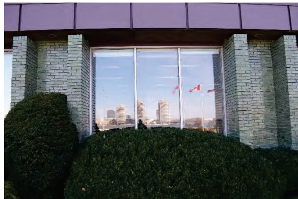
Photo 36: Representative details of bay on north façade, looking south
