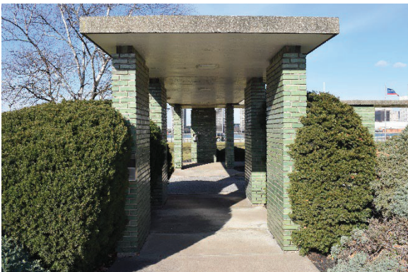
Photo 83: Breezeway south entrance, looking north
