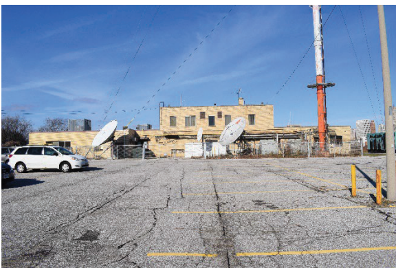
Photo 43: South façade, looking north
