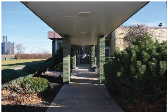
Photo 84: Breezeway, looking east towards main entrance
