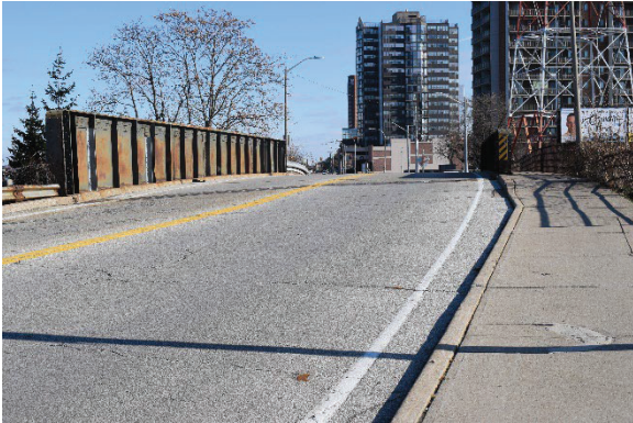
Photo 9: Canadian Pacific Railway Underpass, looking east
