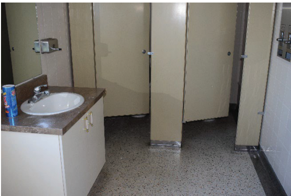
Photo 75: Terrazzo flooring in second storey washroom, looking south
