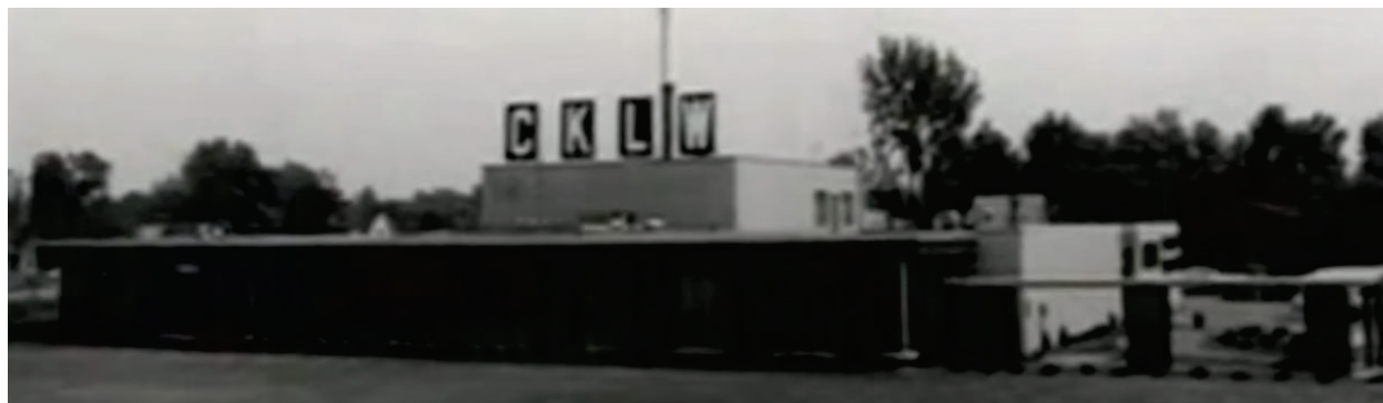
Plate 2 CKLW following completion of Hilliker’s addition (Kryger 2020)
