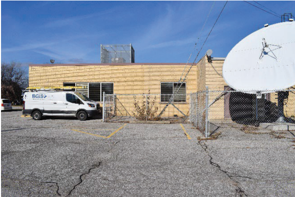
Photo 45: West side of south façade, looking north
