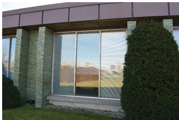
Photo 38: Window details and metal flashing, looking south
