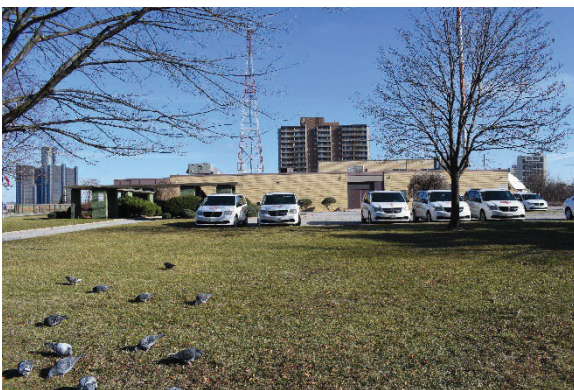
Photo 25: Front (west) façade, looking east
