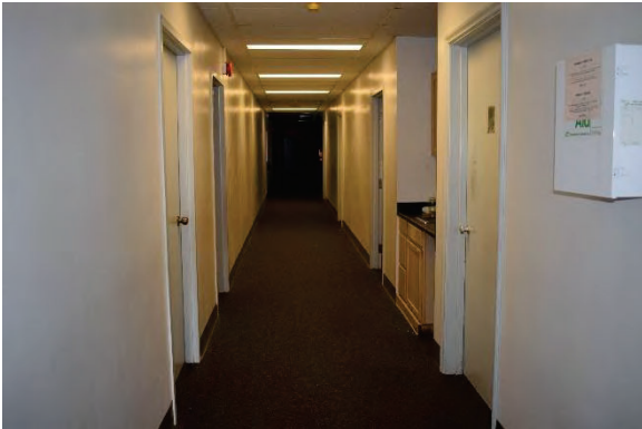
Photo 67: Hallway towards unoccupied area, looking east
