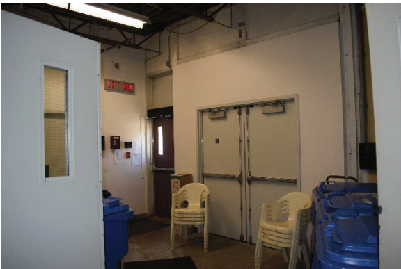
Photo 57: Loading dock, looking west
