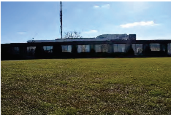
Photo 35: North façade, looking south
