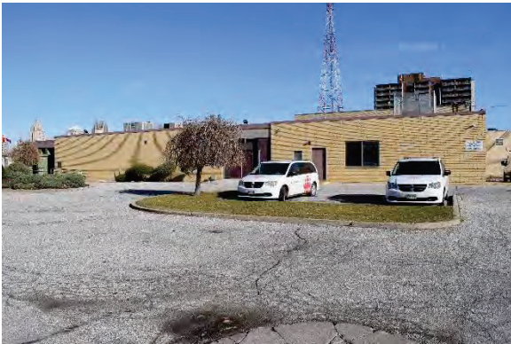
Photo 33: South section of west façade, looking east
