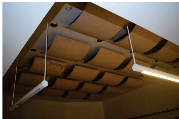
Photo 70: Ceiling with acoustic panels, looking west
