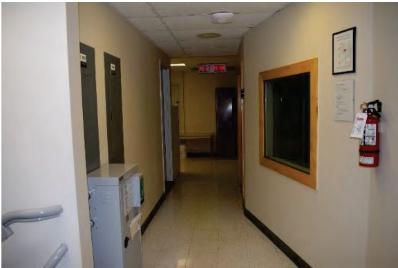
Photo 53: Hallway, looking south
