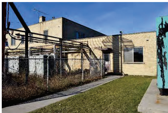
Photo 46: East side of south façade, looking north
