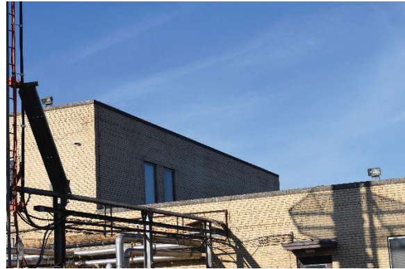
Photo 42: East façade second storey, looking north
