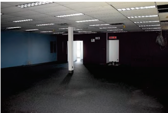
Photo 69: Unused office area, looking east
