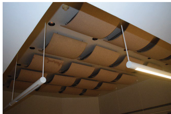
Photo 70: Ceiling with acoustic panels, looking west
