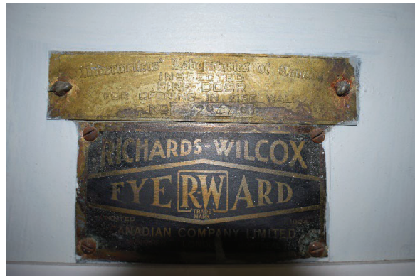
Photo 80: Richards-Wilcox door, looking south
