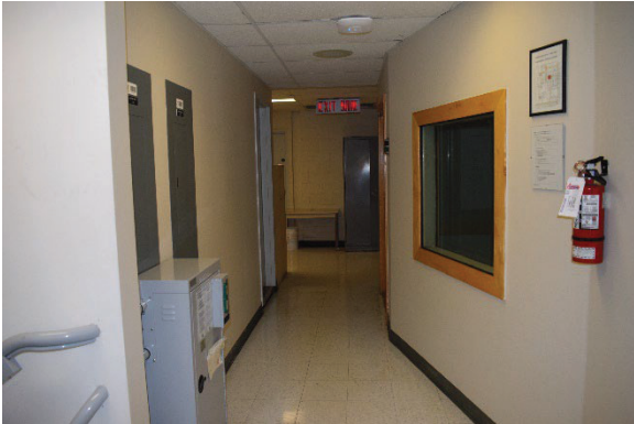
Photo 53: Hallway, looking south
