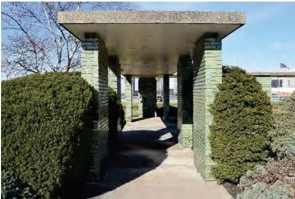
Photo 27: Breezeway south entrance, looking north
