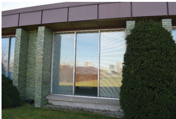
Photo 86: Green glazed brick cladding, looking south.
