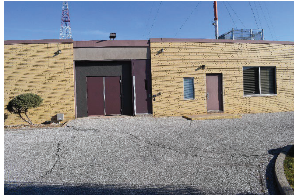
Photo 34: Secondary entrance and windows looking east
