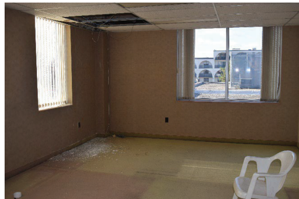
Photo 76: Representative second storey office, looking west
