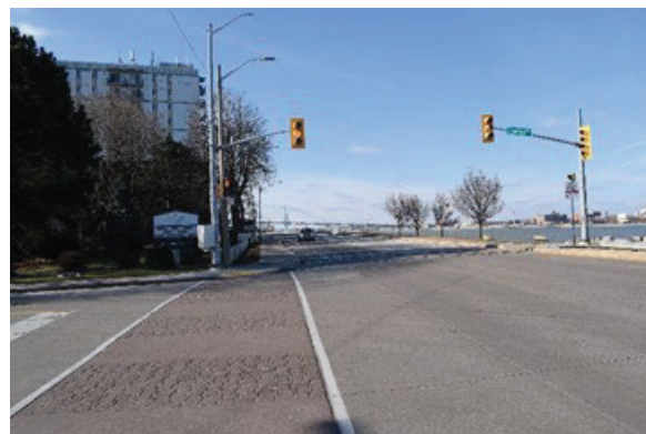
Photo 2: Riverside Drive West, looking west
