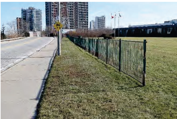
Photo 21: Metal fence, looking east
