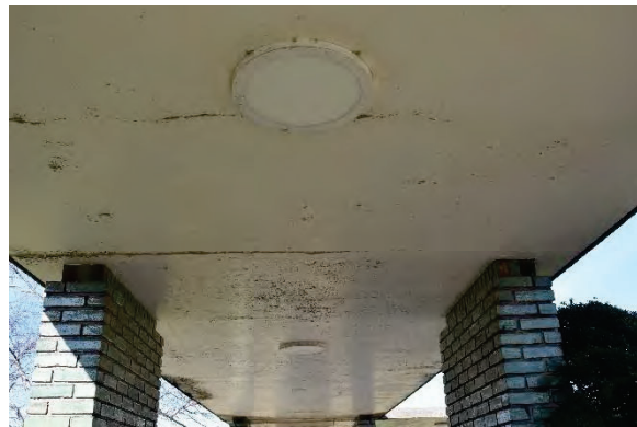
Photo 30: Breezeway ceiling, looking north
