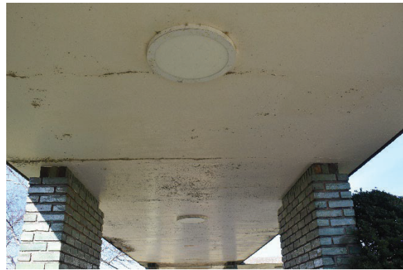
Photo 30: Breezeway ceiling, looking north
