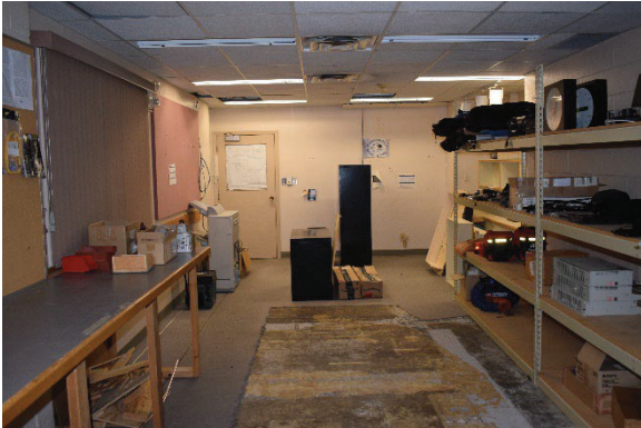
Photo 65: Storage room, representative photo
