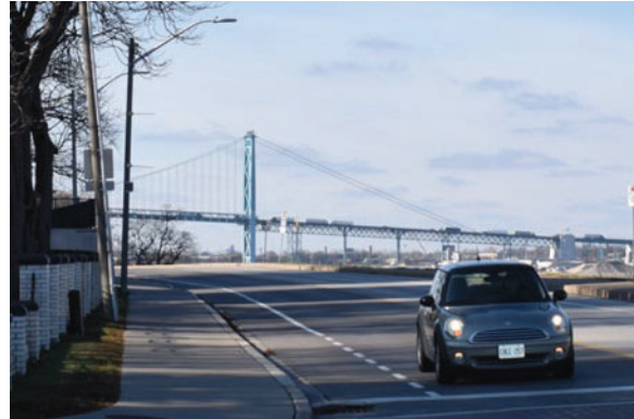
Photo 4: Ambassador Bridge, looking west
