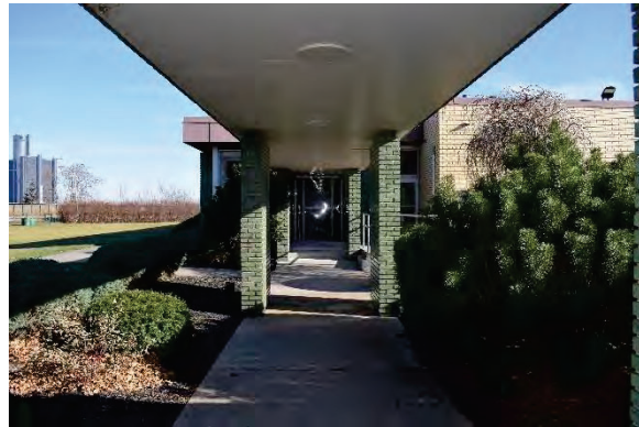
Photo 28: Breezeway, looking east towards main entrance
