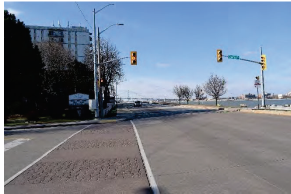
Photo 2: Riverside Drive West, looking west
