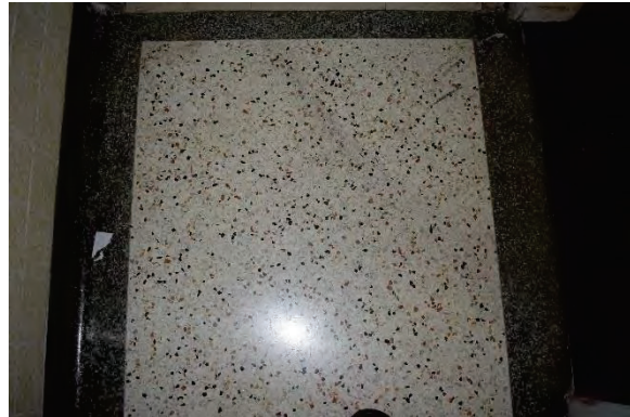
Photo 68: Terrazzo washroom flooring, representative photo
