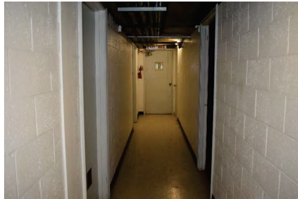
Photo 78: Basement hallway, looking east
