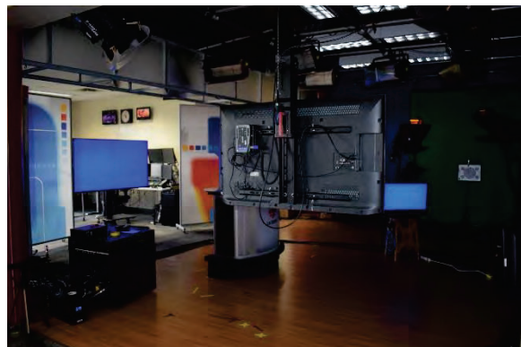
Photo 52: Newscast studio, looking east
