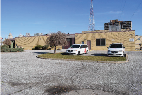
Photo 33: South section of west façade, looking east
