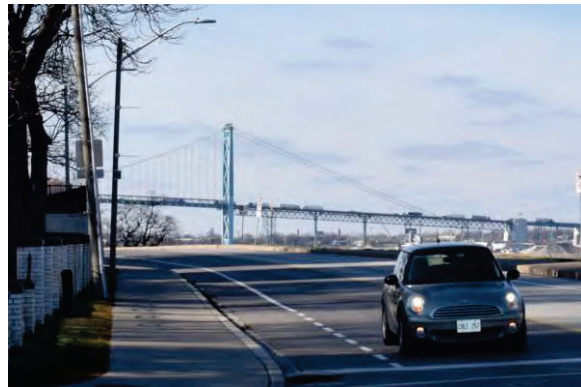
Photo 4: Ambassador Bridge, looking west
