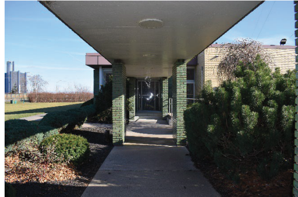
Photo 28: Breezeway, looking east towards main entrance
