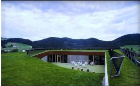
Living Green Roof, with an open air Courtyard & ccessible raised Overlook to view the entire Golf Course
