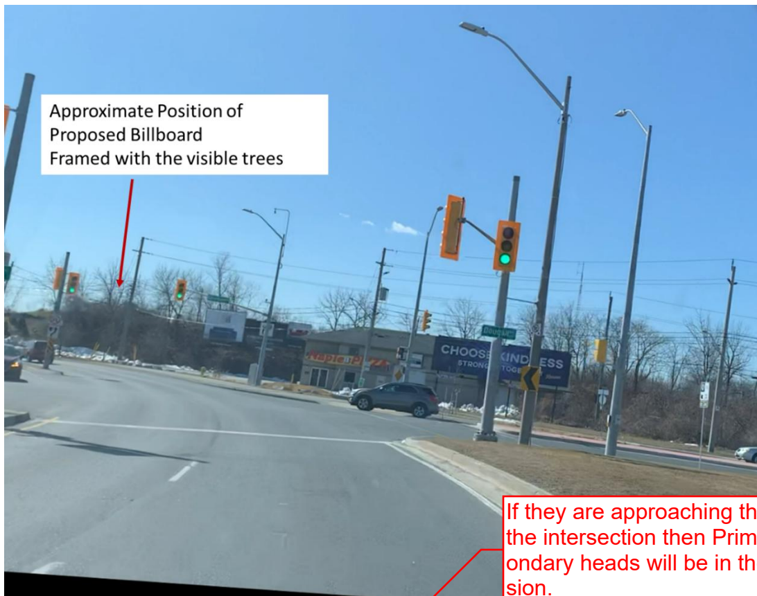
Figure 6: Auxiliary Signal Installed in Southbound Direction
