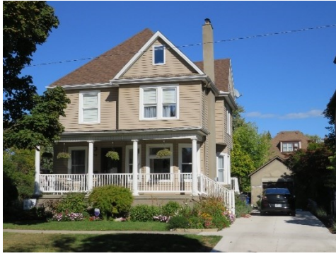
Front (west-facing) facade of 734 Kildare Road, with the detached garage visible at the rear (photo taken by City Staff on October 8, 2025).
