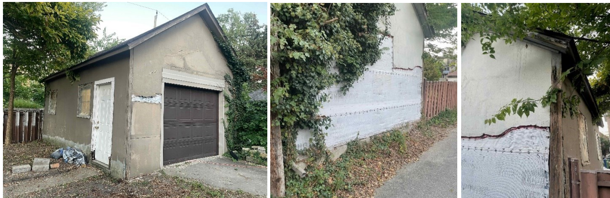
The rear detached garage structure that is proposed to be demolished (photos provided by Property Owners).
