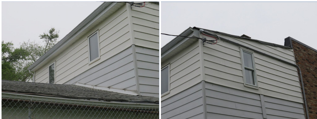
View of the rear two-storey vinyl-clad addition with a sloped shed roof on the commercial building (taken by City Staff on June 6, 2025)
