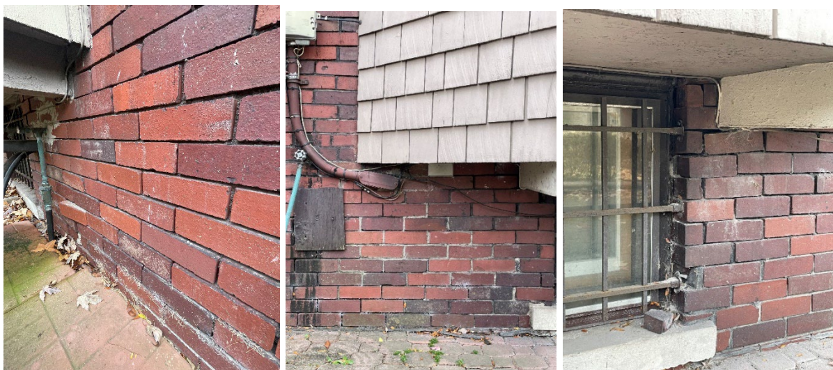
Close-up views of the foundation-level red bricks, showing mortar gaps and loose brick units
