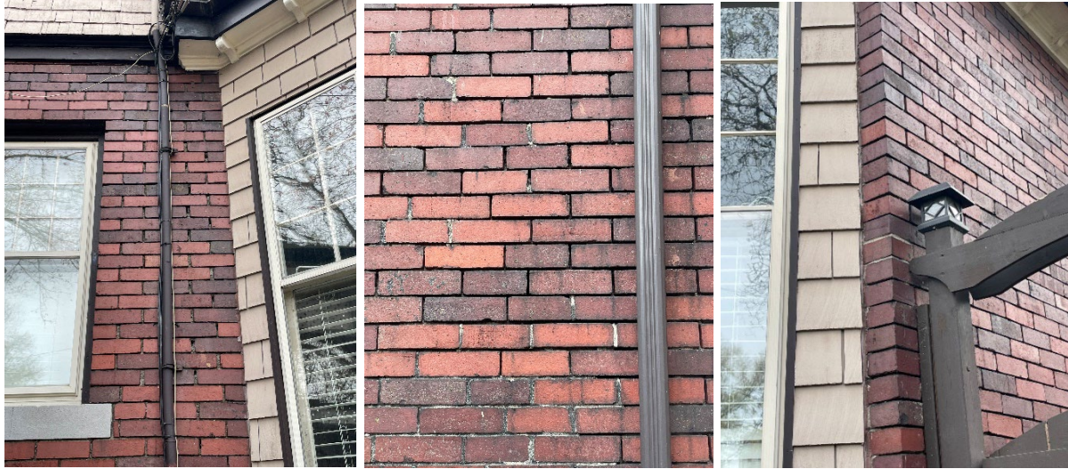
Close-up views of the gaps in the mortar and modern mortar fills on the red brick exterior walls
