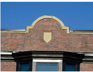
Details of the arched parapet with shield-shaped stone accent and brickwork
