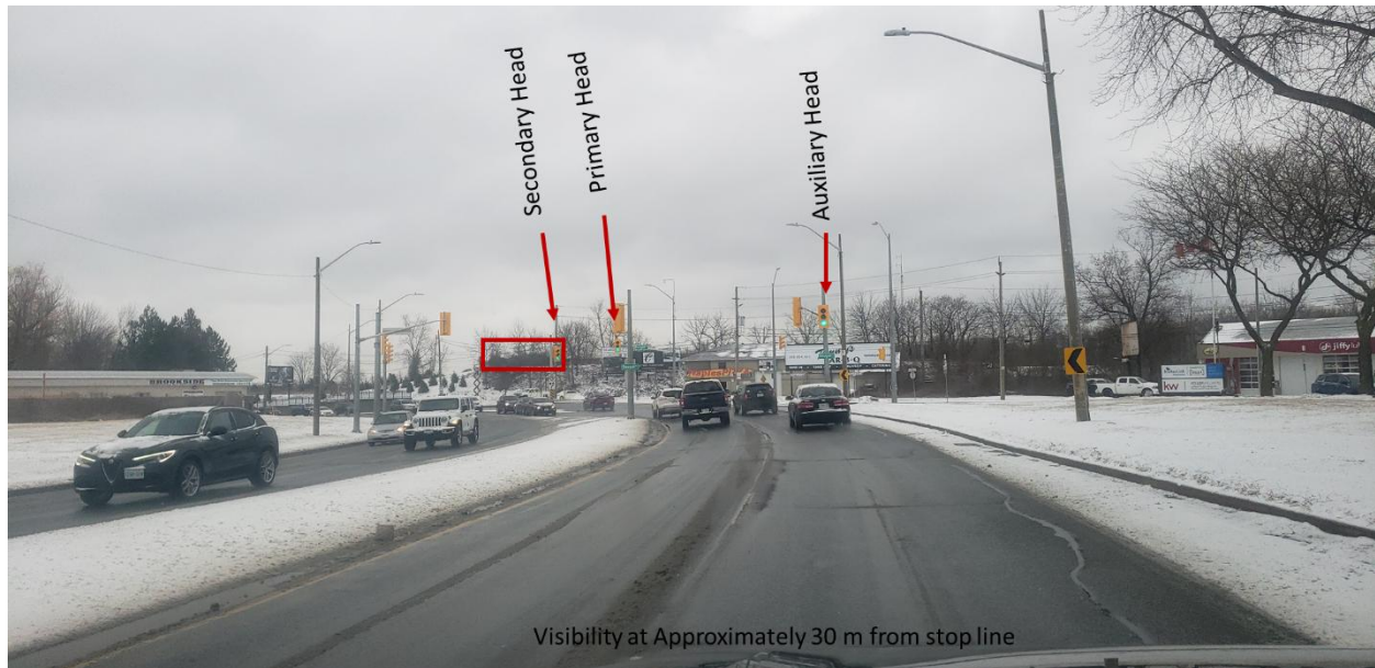
Figure 10: Visibility at 30 m from Stop Line
