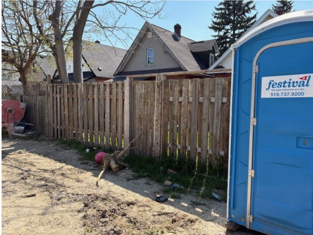
Figure 5 – Rear fence at 1530 Highland
