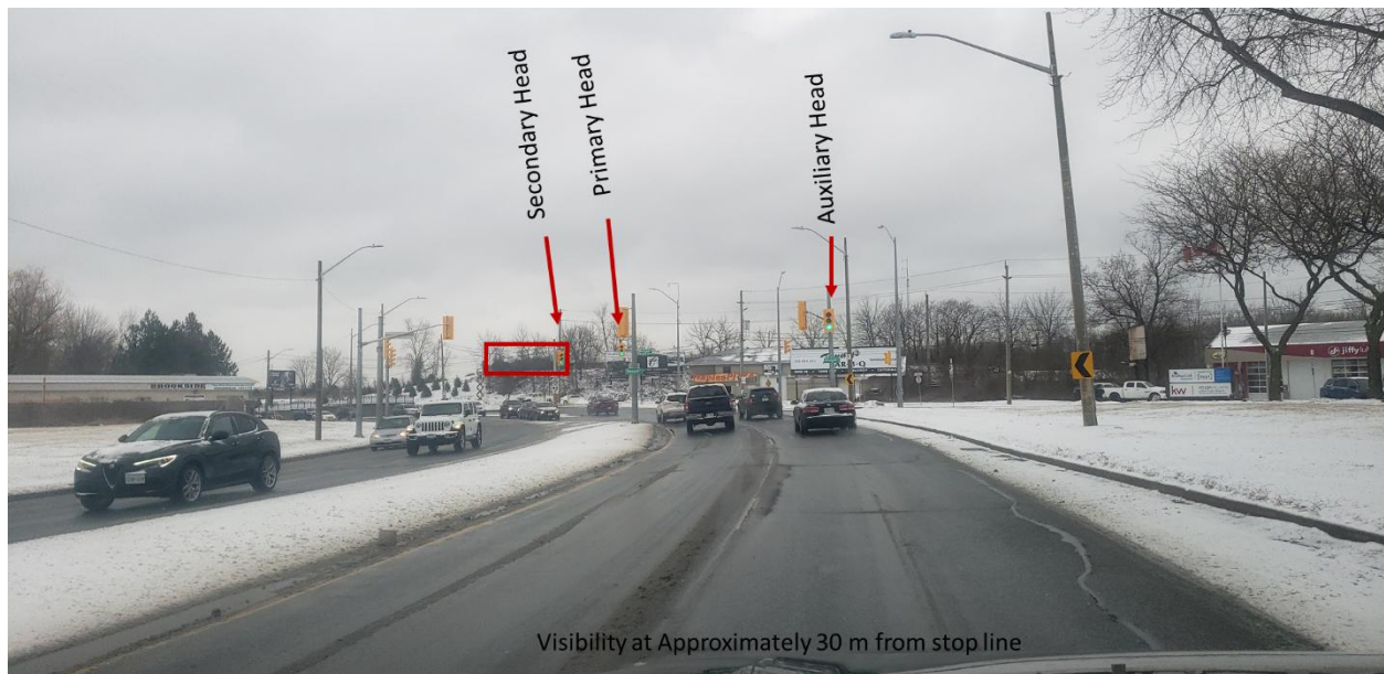
Figure 10: Visibility at 30 m from Stop Line
