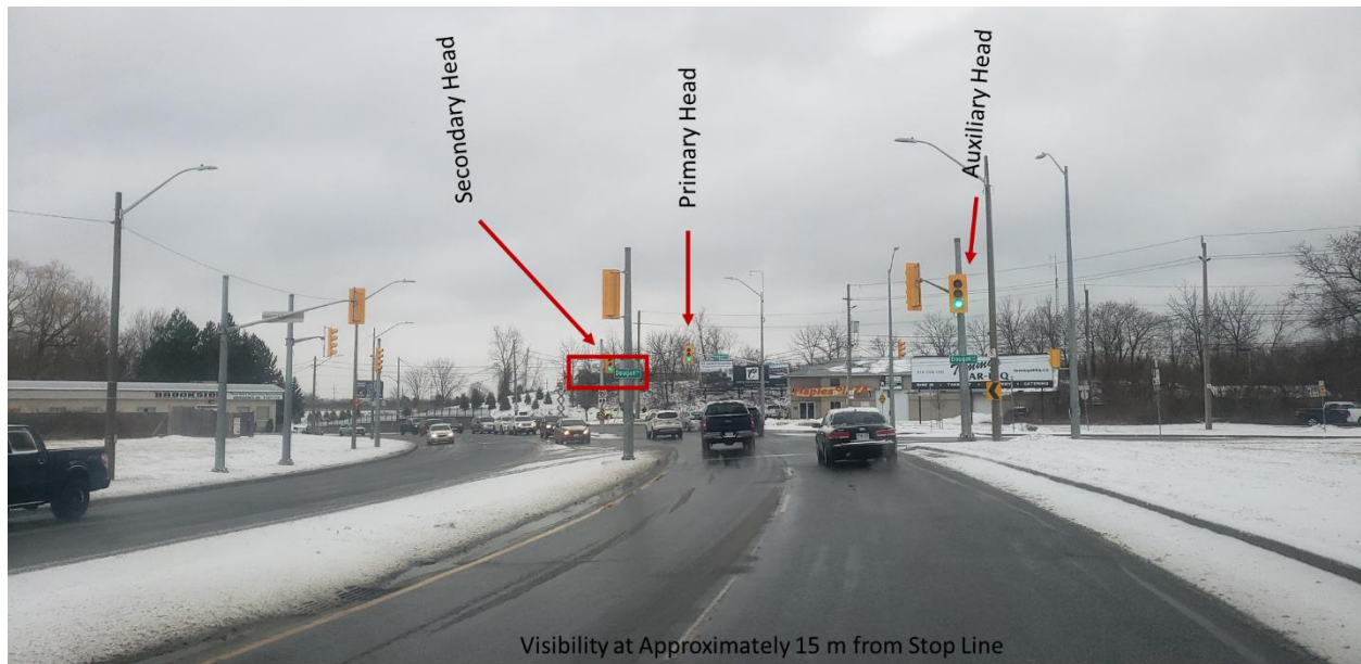
Figure 11: Visibility at 15 m from Stop Line
