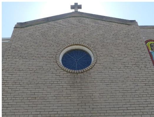
Window detailing on East Elevation
