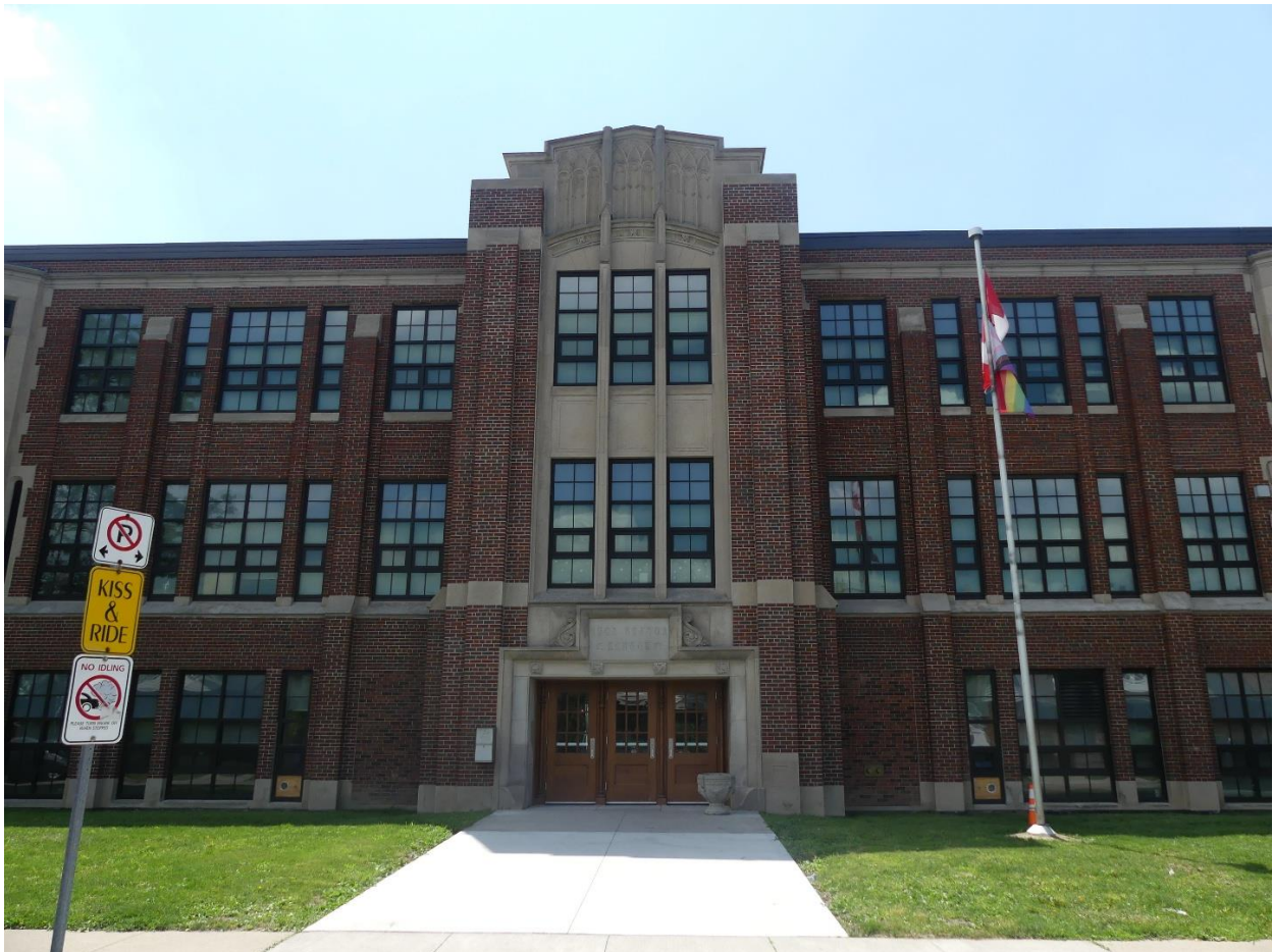
Portion of Front Façade – Site Visit, Heritage Planning Staff (June 2025)
