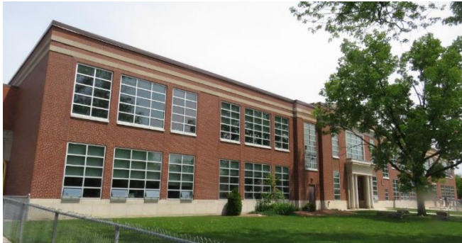
Site Visit, Heritage Planning Staff (May 2025)
