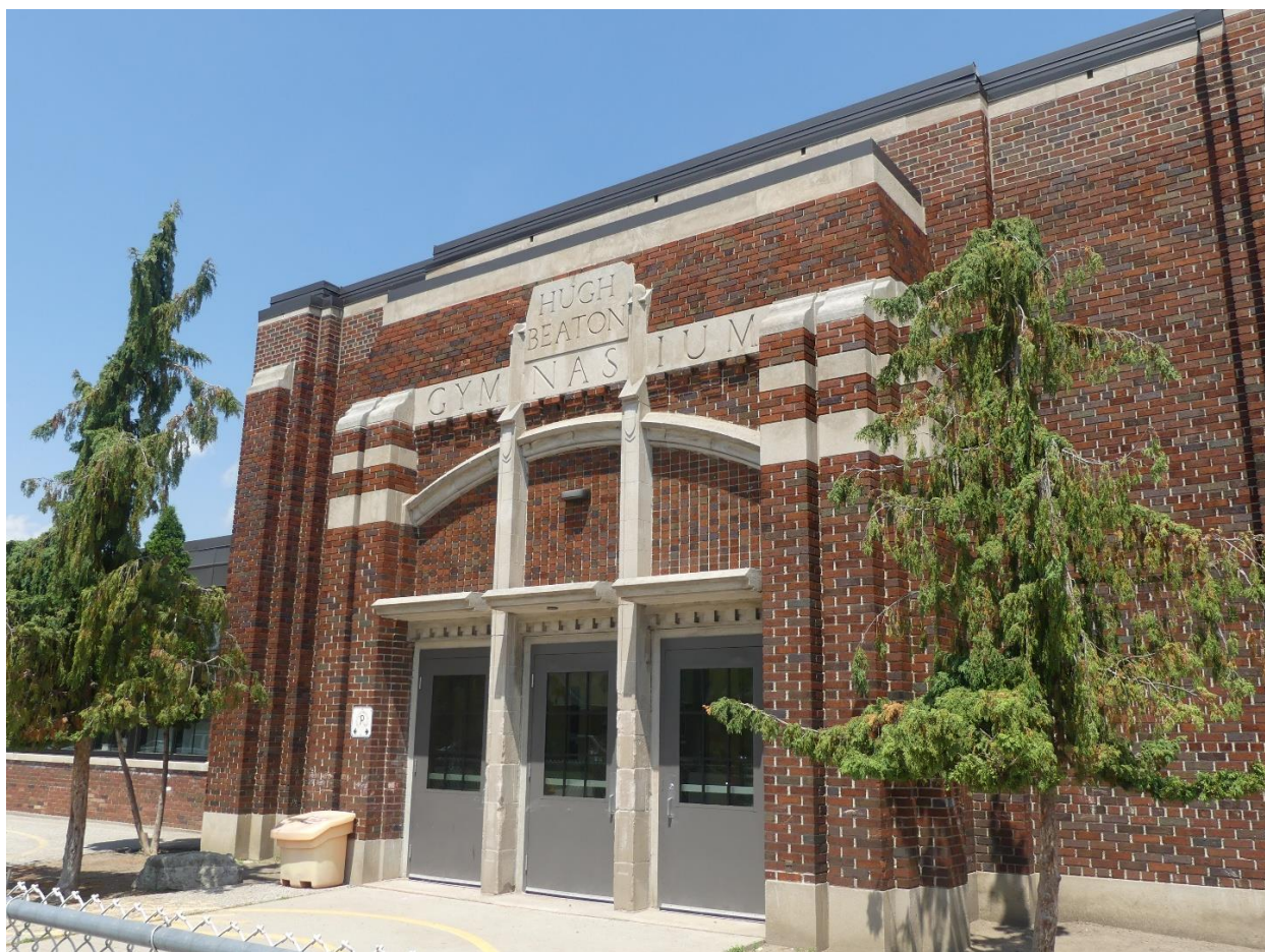
Gymnasium Entrance – Site Visit, Heritage Planning Staff (June 2025)
