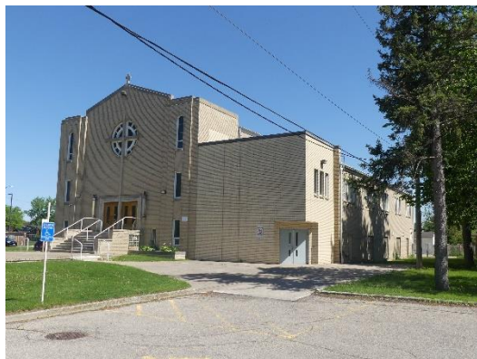
North and West Elevations
