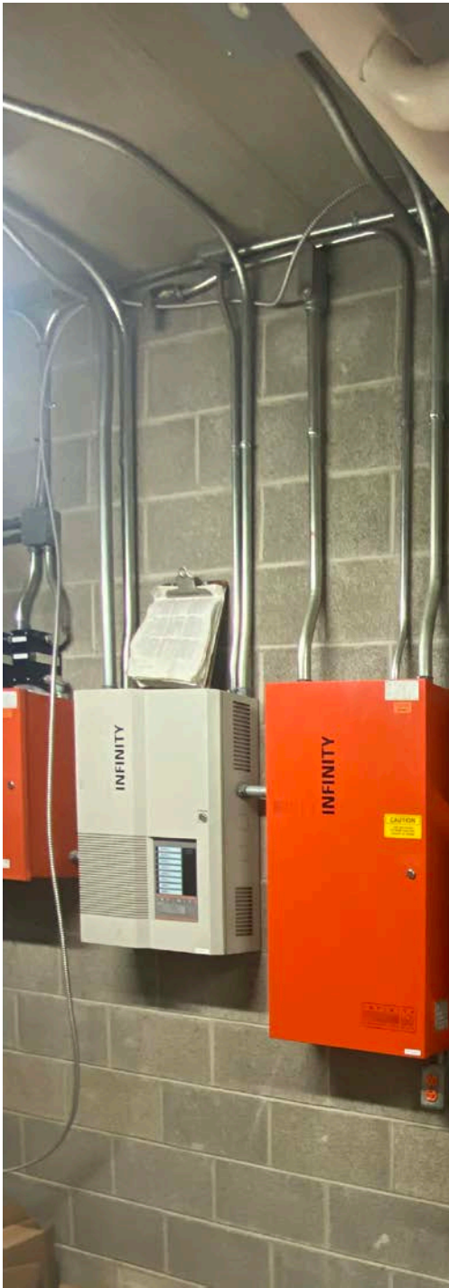
Figure 1-9 New Intercom / Interphone System at 920 Ouellette Completed in 2024
