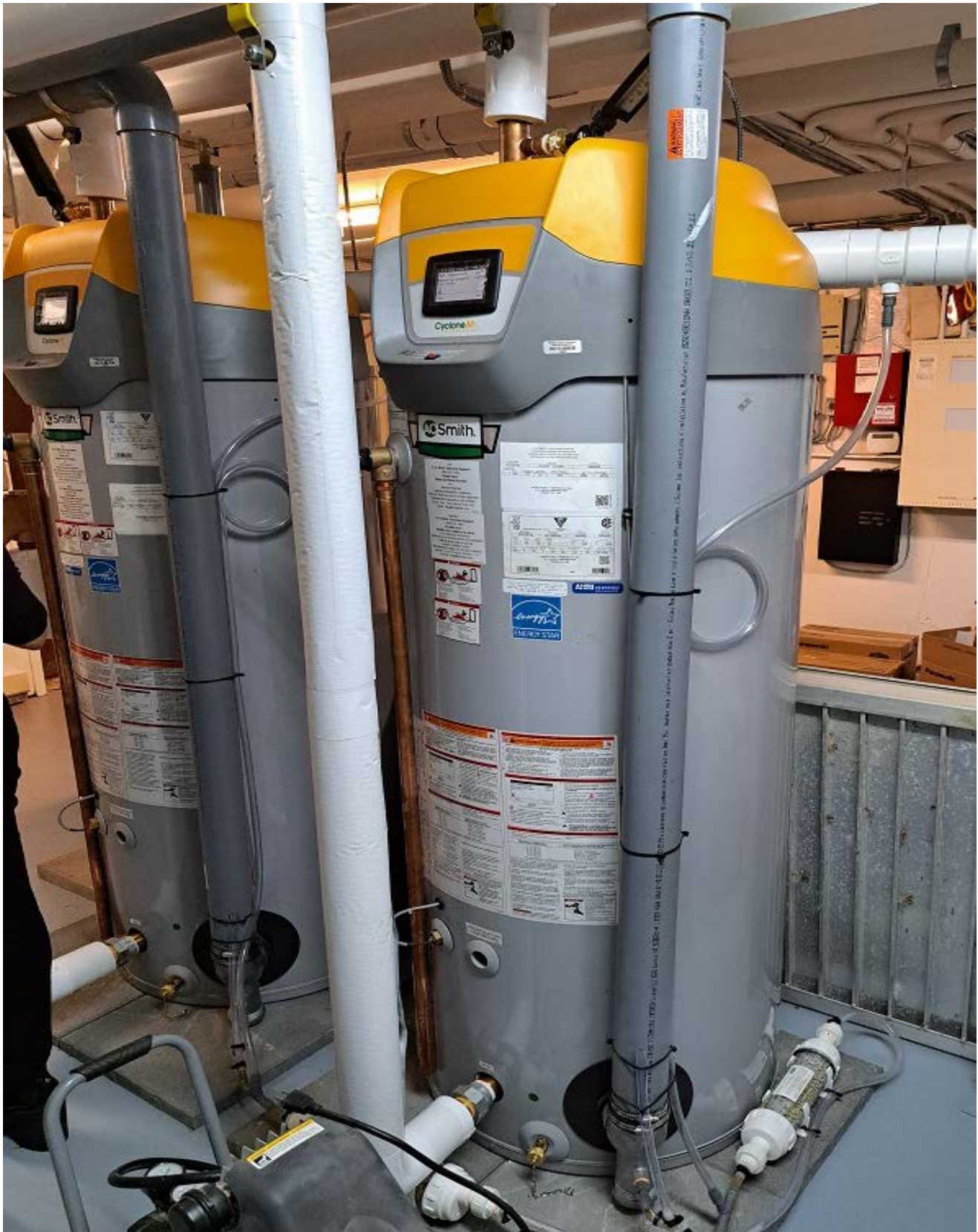
Figure 1-7 New Condensing Gas Powered Domestic Hot Water Tank High Efficiency Completed in 2024
