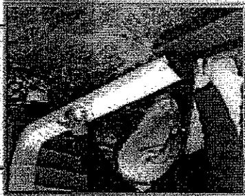
• A downspout pipe extension is attached. A splash board may be used to prevent erosion.
