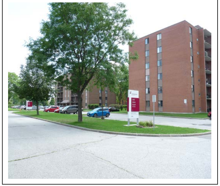
St. View – looking SW at 1145 & 1175 Adair Ct
