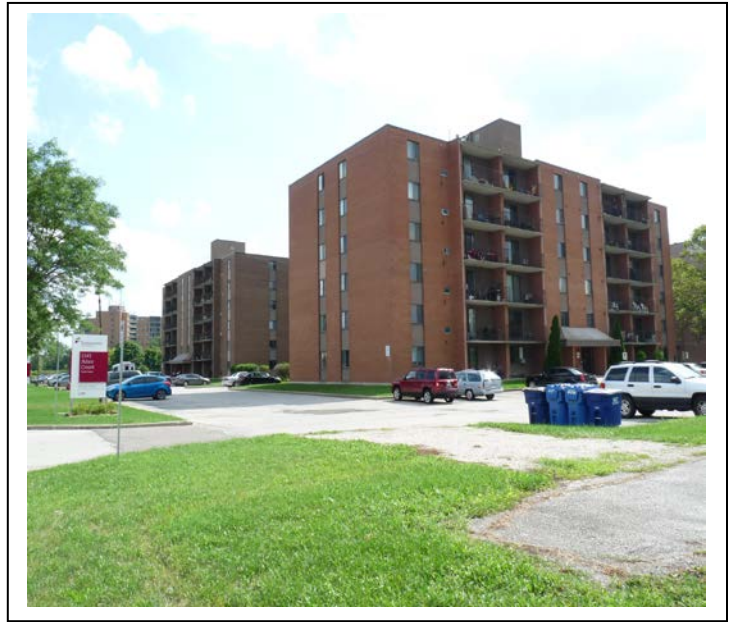
St. View – looking SW at front of 1145 Adair Ct
