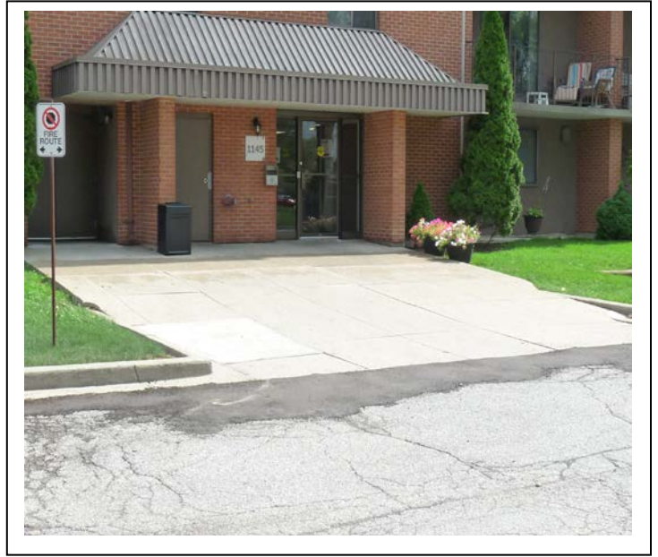
Parking Area View – looking south at main entrance
