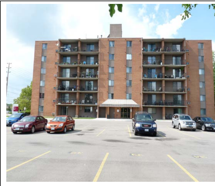
Street View – looking N in south side building
