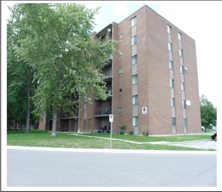
Parking area view – SW corner of 1175 Adair Ct building
