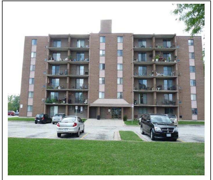
St. View – looking west at front of building
