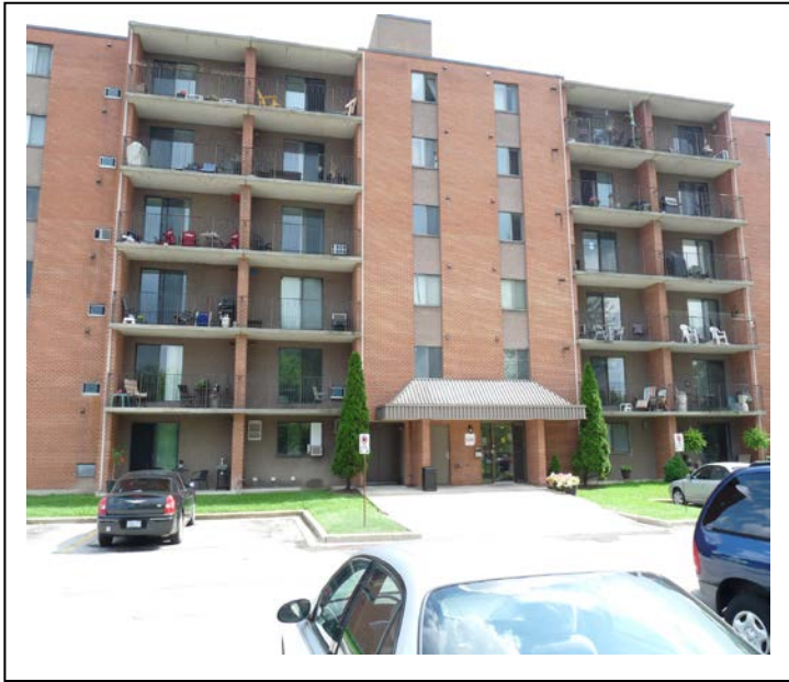
Parking Area View – looking S at north side 1145 Adair Ct
