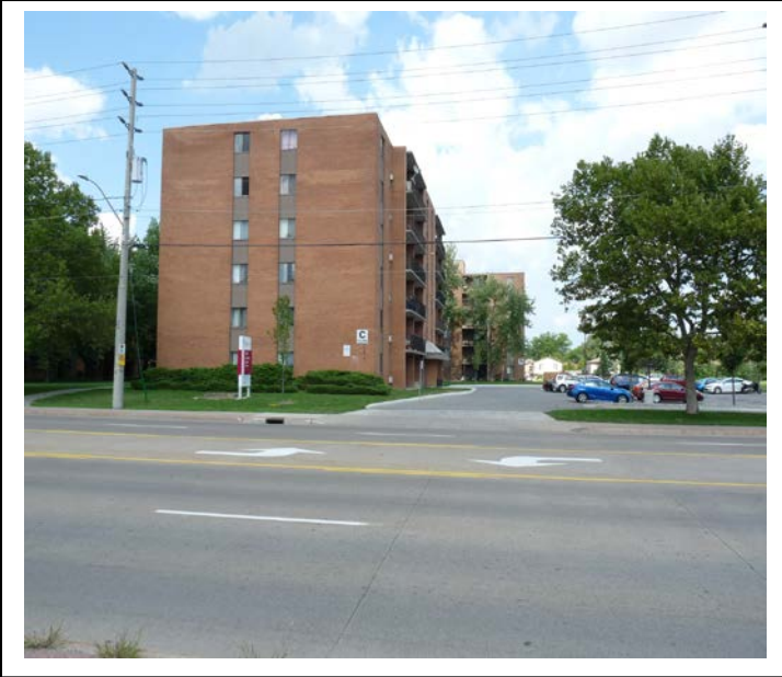
Street View – looking East at west side of building
