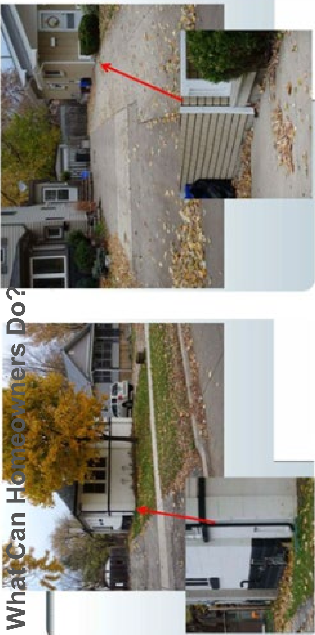
Disconnected Downspout
