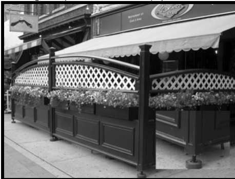
Alternative post attachment with no direct anchoring
