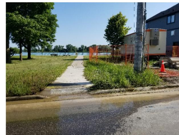
**8717 RIVERSIDE DRIVE** – Water level elevation of 175.6m on Aug 2<sup>nd</sup>. Observed water flowing onto Riverside Drive from storm sewer manhole. This manhole is connected with outfall from 8717 Riverside Drive to the Detroit River.
