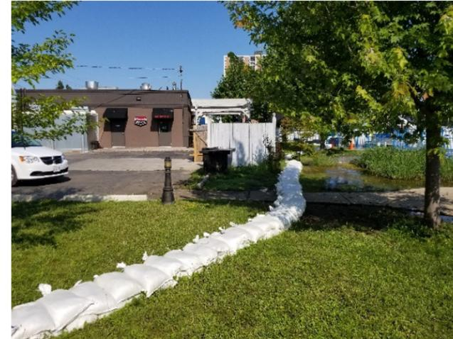
**LAKEVIEW MARINA** – Water level elevation of 175.6m on Aug 2<sup>nd</sup>. Observed pooling of water in the area between Armando’s Pizzeria and the sheet piles boundary of the marina. Sandbagging in place limits flooding to this immediate area, but if allowed to flow freely, overland flow at this location would reach Riverside Drive and flow down Riverdale Ave.
