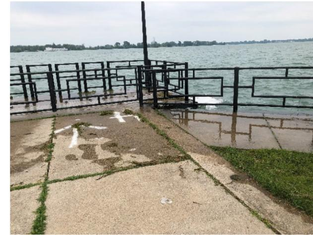
**ST. ROSE BEACH** – Water level elevation of 175.7m on July 7<sup>th</sup>. Observed shallow waves overtopping pedestrian walkway and spilling water and debris onto Riverside Drive.
