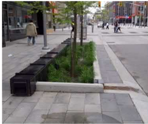
Bioretention Planter (Kitchener, ON)
