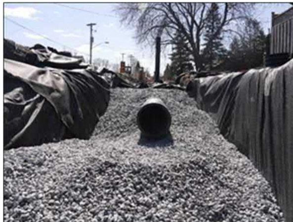
Perforated pipe installation (Mississauga, ON)
