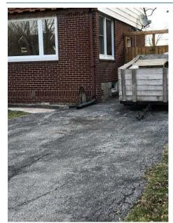
Photo 10: Disconnected Downspout
