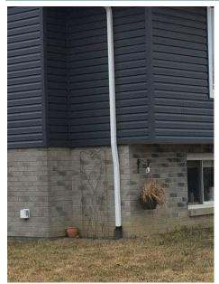
Photo 43: Connected Downspout
