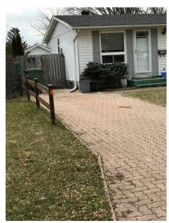
Photo 3: Disconnected Downspout
