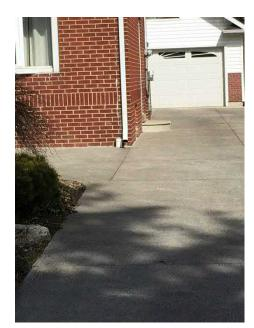
Photo 51: Disconnected Downspout
