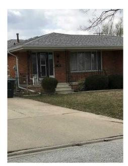
Photo 6: Disconnected Downspout
