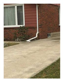
Photo 48: Disconnected Downspout
