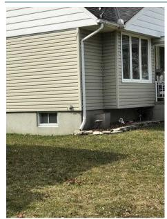
Photo 22: Disconnected Downspout
