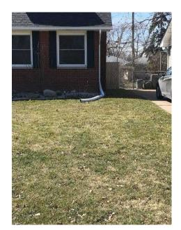
Photo 33: Disconnected Downspout
