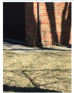
Photo 37: Connected Downspout
