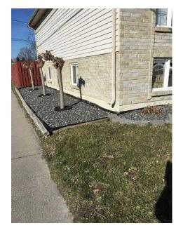
Photo 42: Disconnected Downspout
