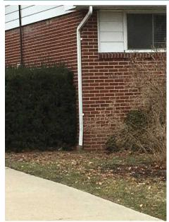
Photo 46: Connected Downspout
