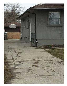
Photo 30: Disconnected Downspout
