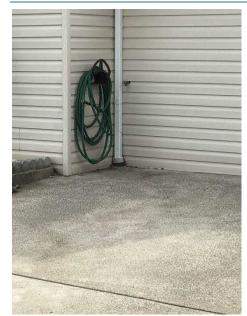
Photo 19: Connected Downspout
