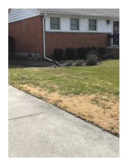
Photo 18: Disconnected Downspout
