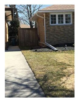
Photo 39: Disconnected Downspout
