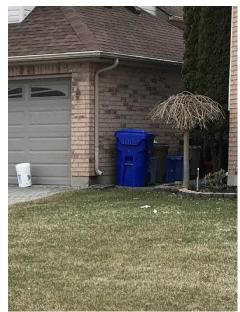
Photo 7: Disconnected Downspout
