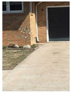
Photo 31: Connected Downspout
