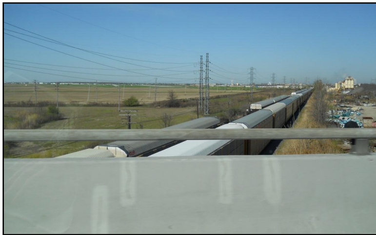
Figure 8 - Lauzon Parkway Bridge over CPR
