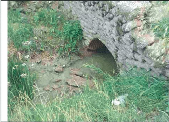
Photograph 13 ↑ Lachance Drain – East side of Banwell Road, culvert
