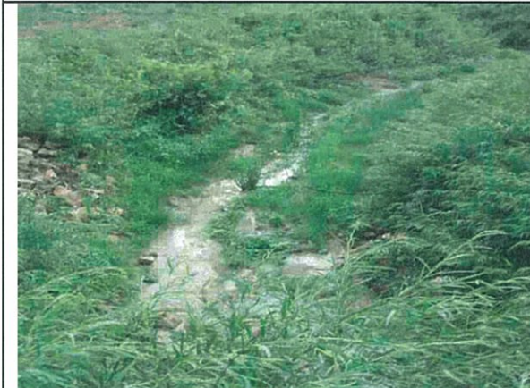
Photograph 15 ↑ Lachance Drain – West side of Banwell Road, looking west
