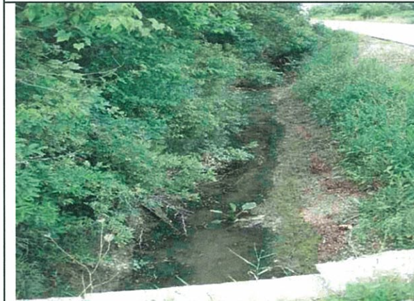
Photograph 11 ↑ Gouin Drain – West side of Banwell Road, looking west
