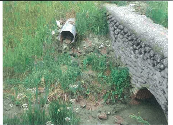
Photograph 14 ↑ Lachance Drain – East side of Banwell Road, drainage pipe and culvert
