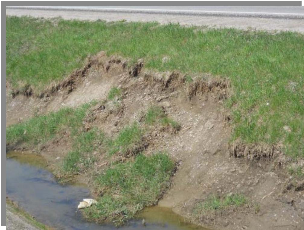
PLC3-3 Erosion on Channel Slope Just North of Culvert
