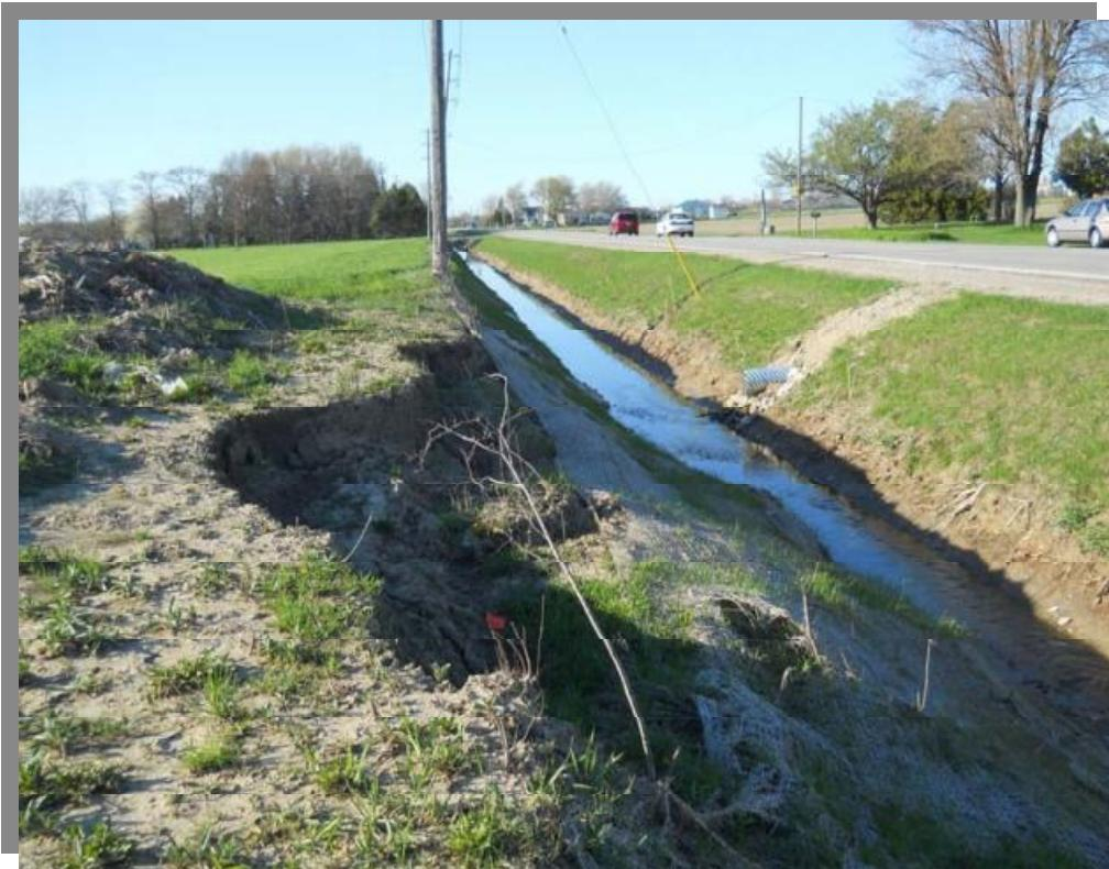
PLC10-4 West Channel Bank Failure (Watson Drain - Looking North)
