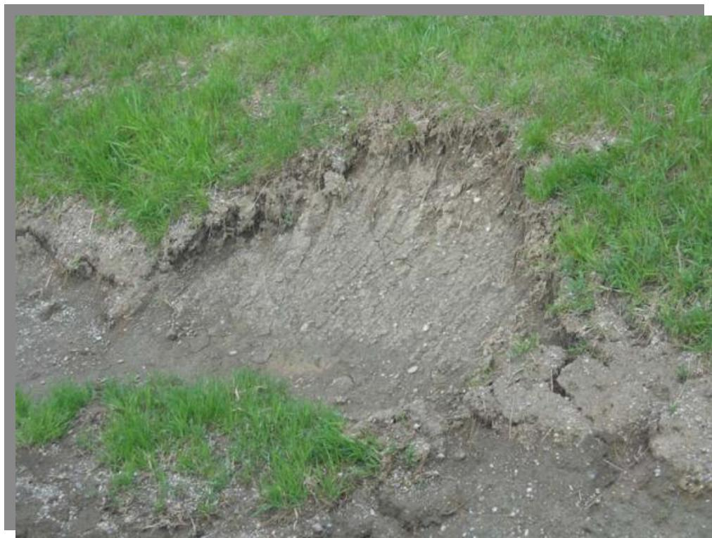
PLC2-4 Erosion on Channel Slope (Just north of Culvert LC2)
