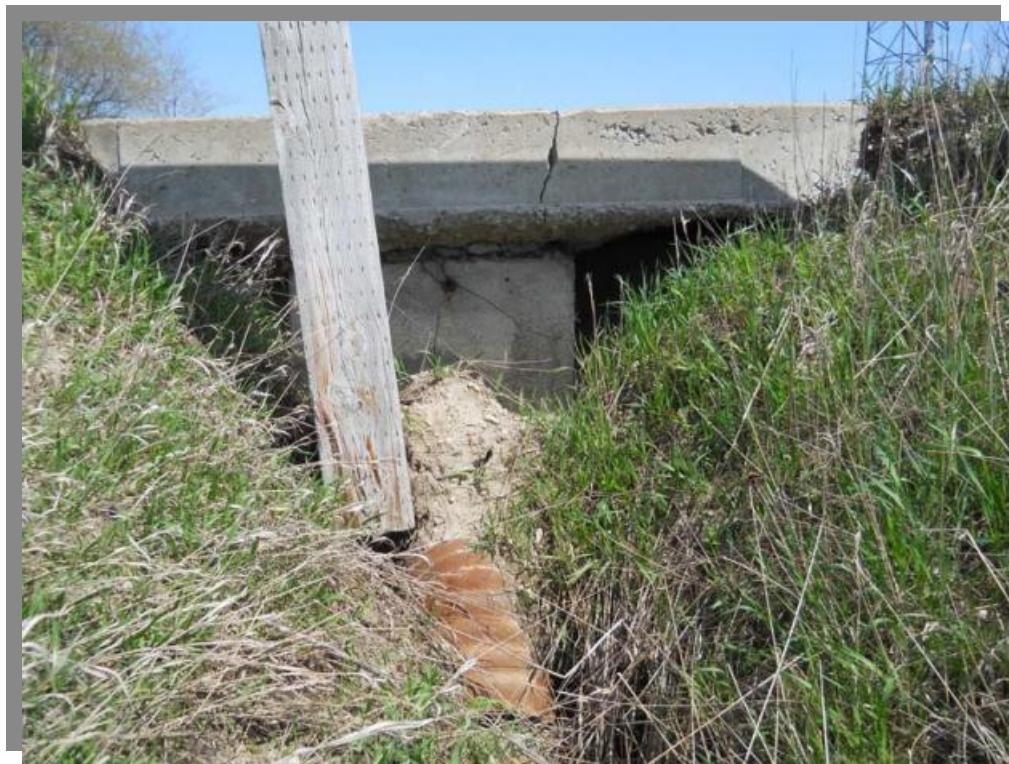
PS-2 Looking at Exposed CB, CSP Pipe and Wood Guardrail Post
