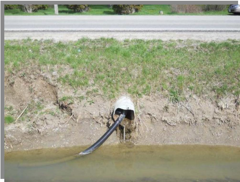
PLC4-1 Downstream Elevation (Erosion on channel slope)
