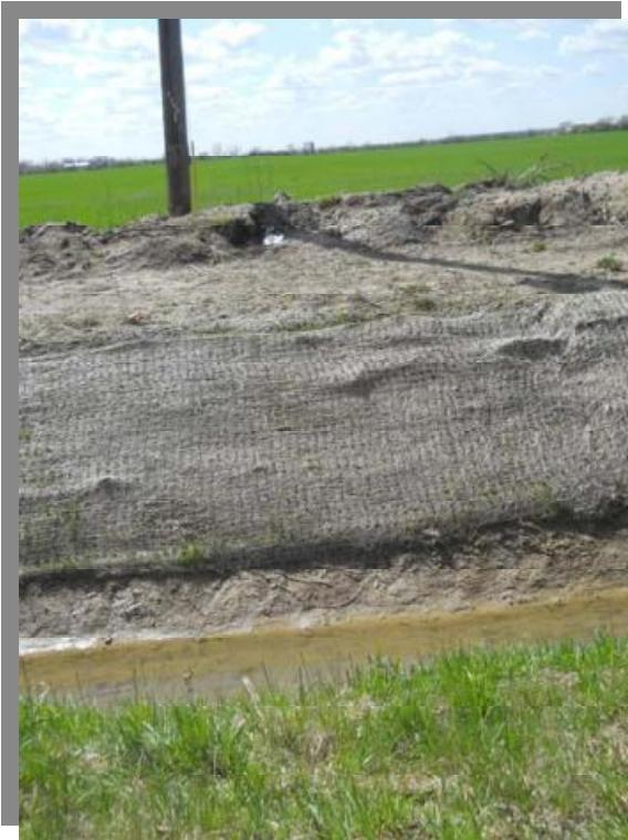
PLC2-3 Insufficient Blanket Protection on West Channel Bank
