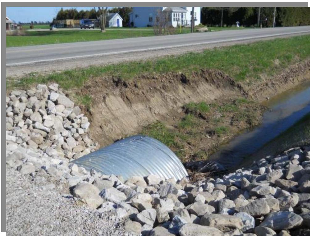
PLC7-5 Erosion on East Channel Slope Upstream of 1800mm CSP (65m± north of Culvert LC7)
