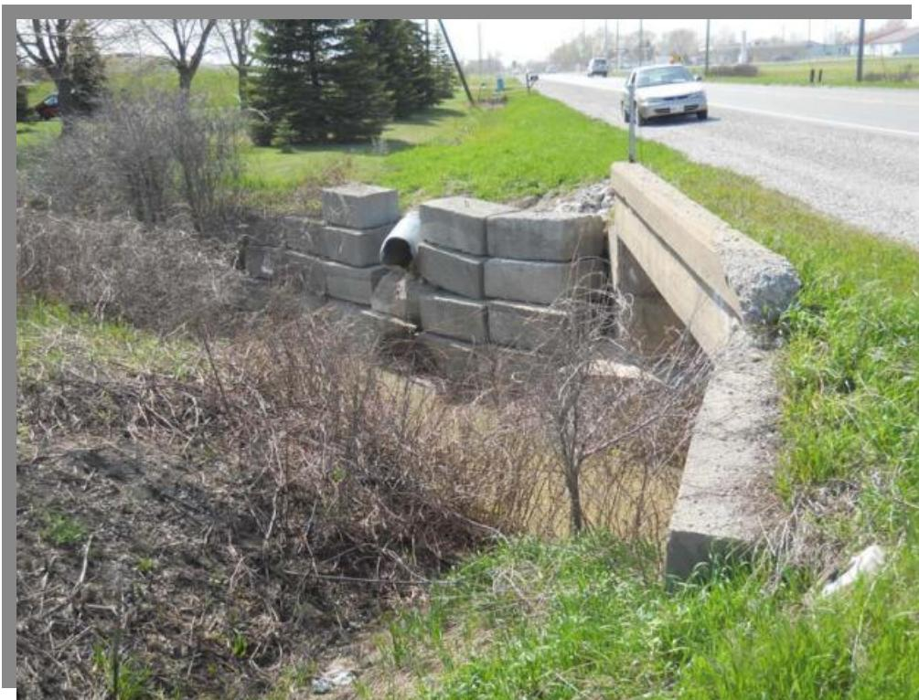
PDC5-4 Upstream Elevation (Spalling at east end of top beam)
