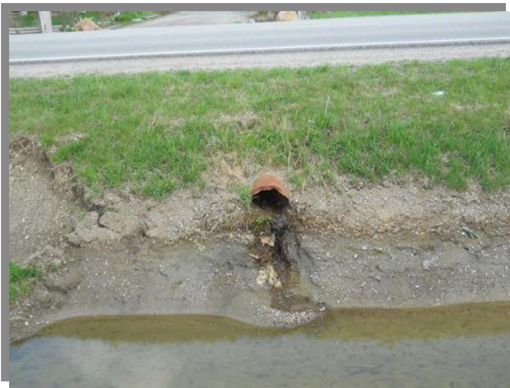
PLC2-1 Downstream Elevation (Erosion on channel slope)
