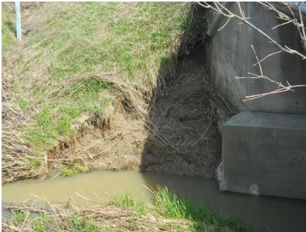
PDC5-2 Erosion Adjacent to East Culvert Footing (Downstream side)
