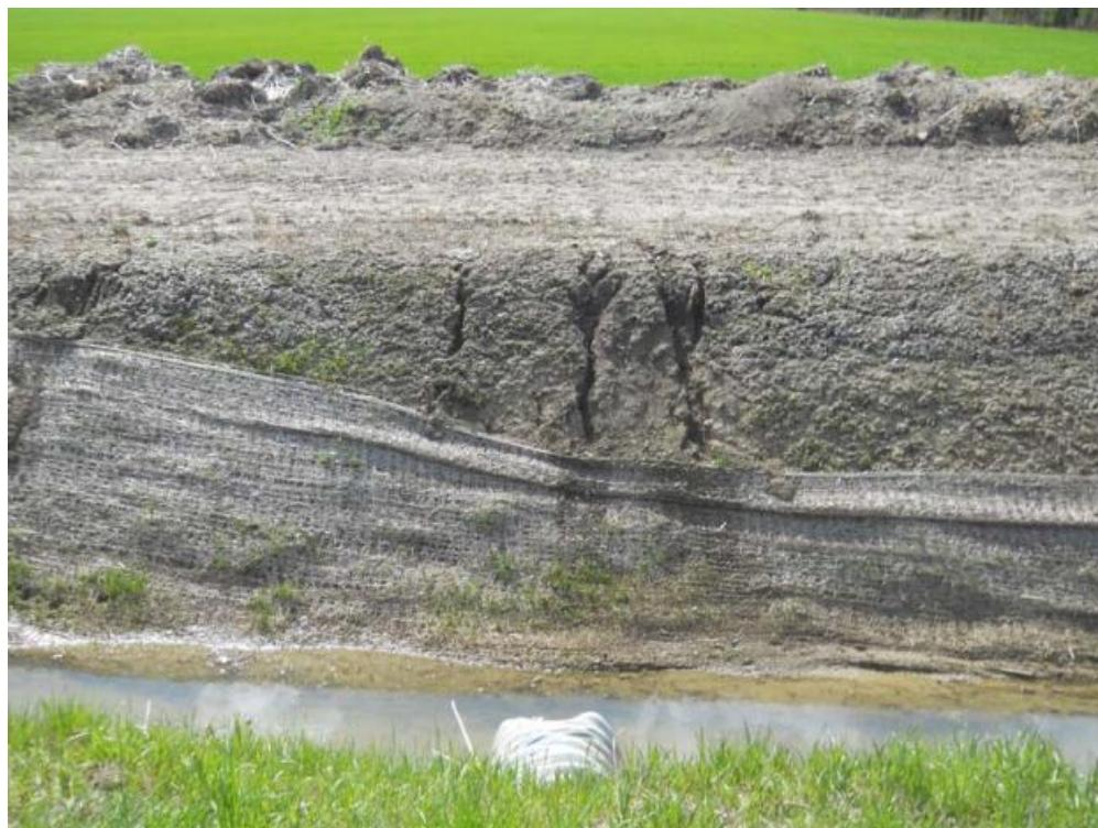
PLC4-4 Erosion Blanket Failure (West channel slope)
