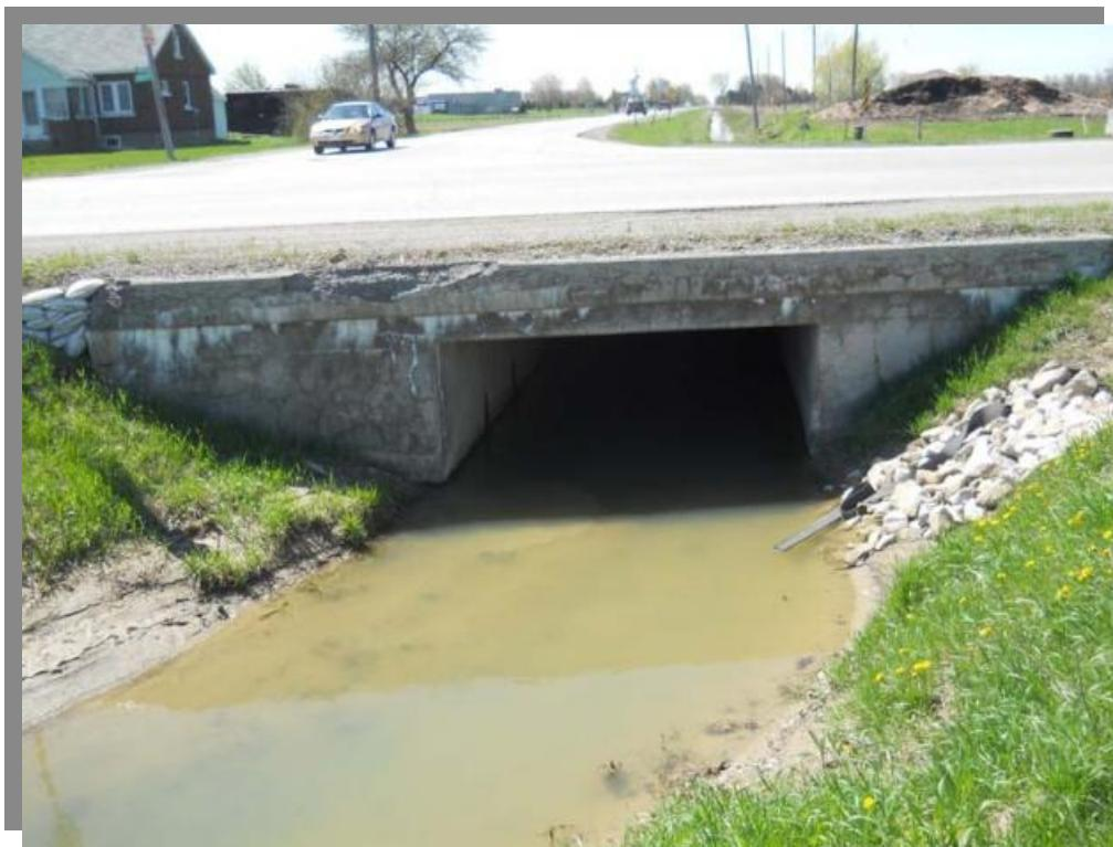
PDC2-1 Downstream Elevation (Spalling at top of culvert-Watson Drain)
