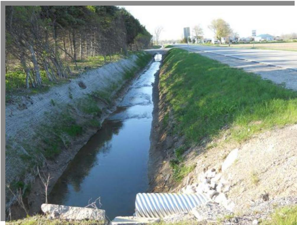
PLC11-3 Deteriorated Erosion Blanket on West Channel Slope (Watson Drain)
