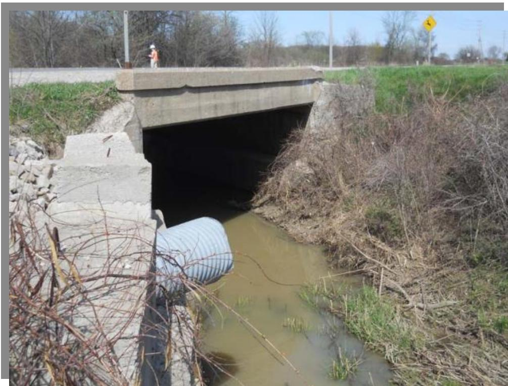
PDC5-3 Upstream Elevation (Spalling on top of culvert left corner)
