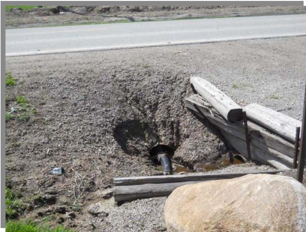
PLC2-2 Upstream Elevation (Erosion above pipe)
