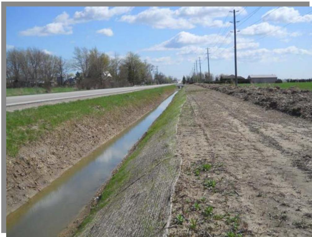
PLC3-4 Insufficient Blanket Protection on West Channel Bank (Looking south)
