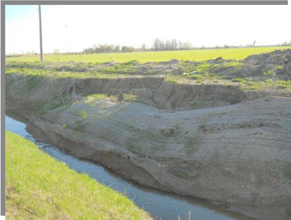
PLC10-3 West Channel Bank Failure (Watson Drain)
