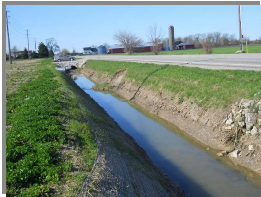
LC7-6 Erosion on East Channel Slope (Opposite side of tiled system outlet pipe)
