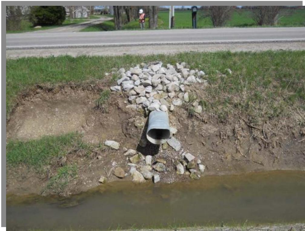
PLC3-1 Downstream Elevation (Erosion on channel slope)
