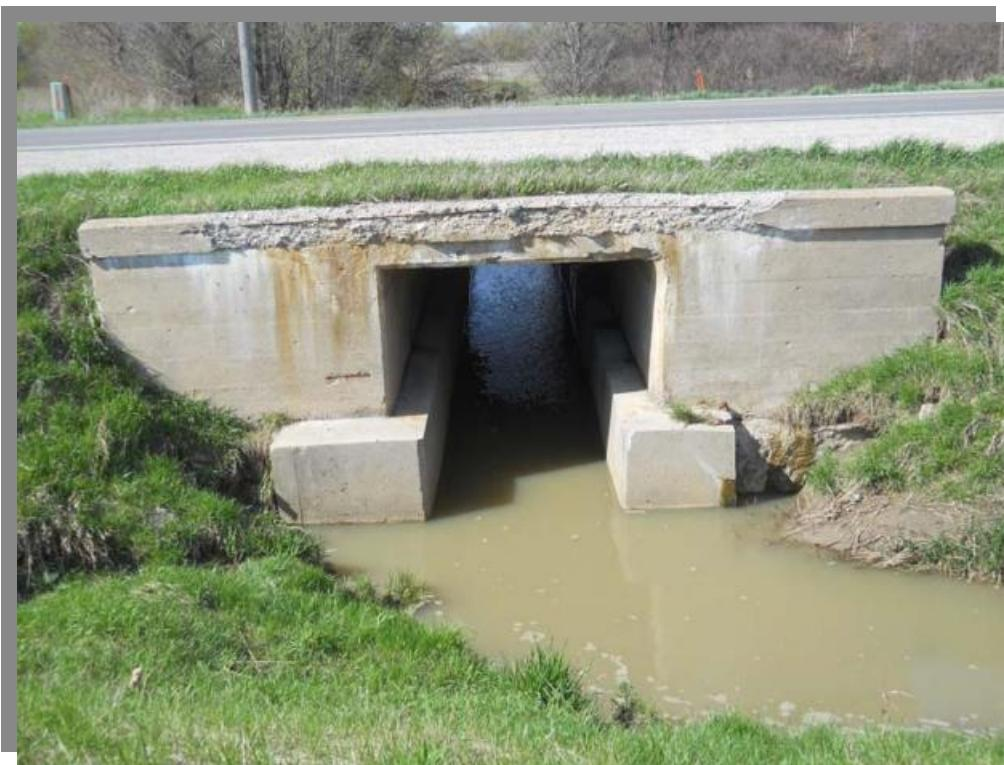
PDC6-2 Upstream Elevation (Spalling and exposed rebar on top of culvert)
