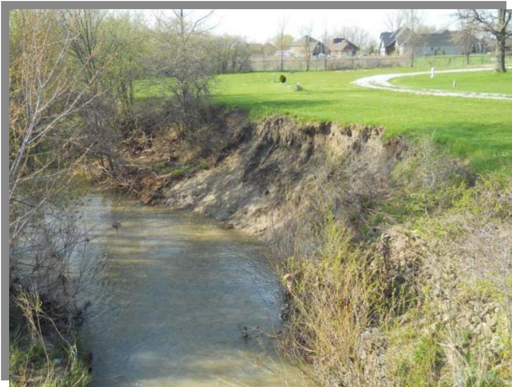
PDB2-3 Erosion on East Bank (Downstream side – Looking north)
