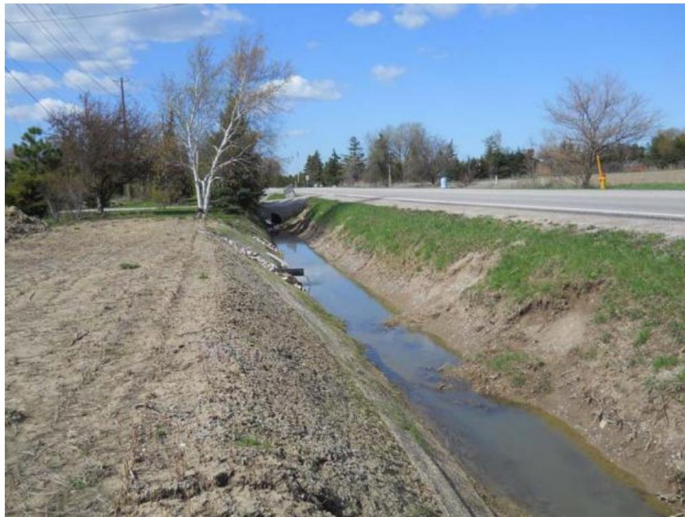
PLC4-3 Erosion on East Channel Slope and Erosion Blanket Failure (Looking north)
