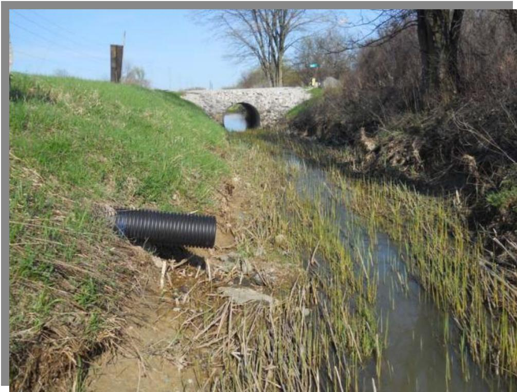
PDC7-3 Erosion on Bottom of Channel Bank (Looking east)
