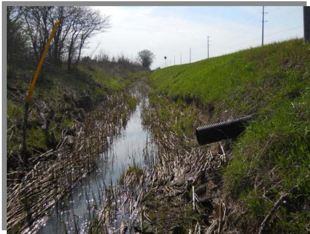
PDC7-2 Erosion on Bottom of Channel Bank (Looking west)
