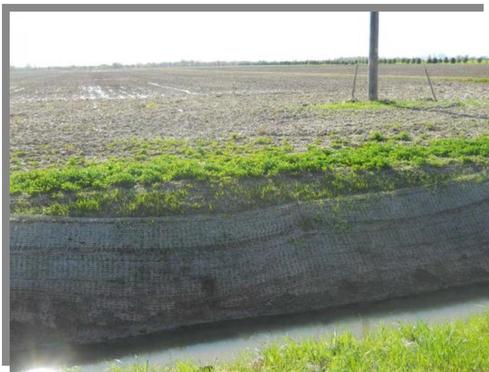
PLC7-4 Erosion Blanket Failure (West channel slope)
