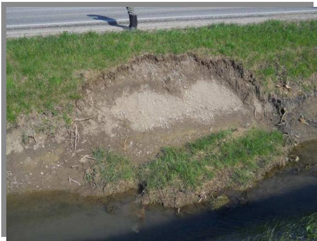
PLC7-3 Erosion on East Channel Slope
