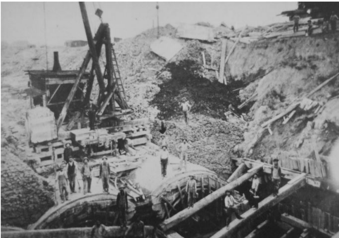
Figure 3.3.3b: Tunnel construction, cut and box method, with tunnel section in foreground and steep banks on the right, Windsor side. From Hiram Walker Museum Collection (Tennant 1991:124).
