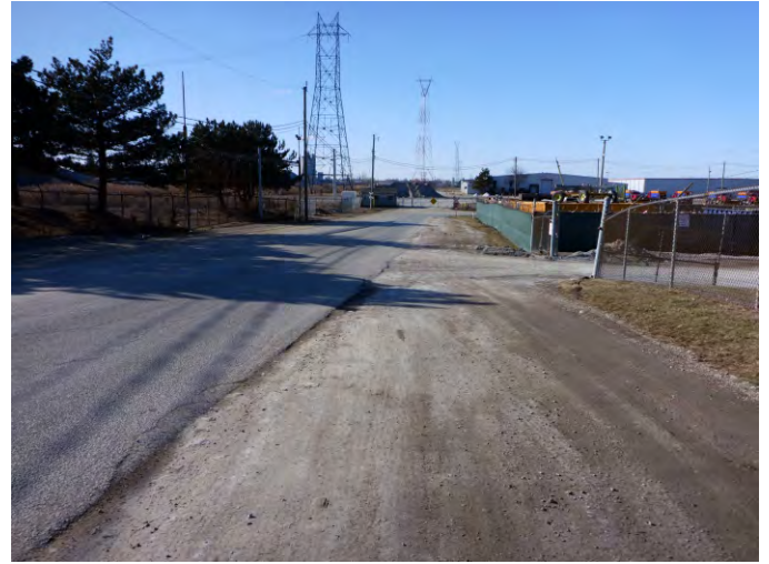
Plate 3.1-2: Prince Rd Sewer Outfall - Looking west along Chappell Ave. towards Russell St. and the industrial yard within the Study Area. (Photo P1020117).
