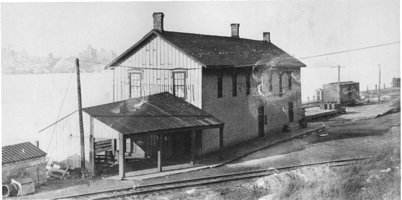
Figure 3.3.3a: Canada Southern Railway Station, Windsor; adjacent to the ferry slip on Cameron Avenue (Tennant 1991:130).
