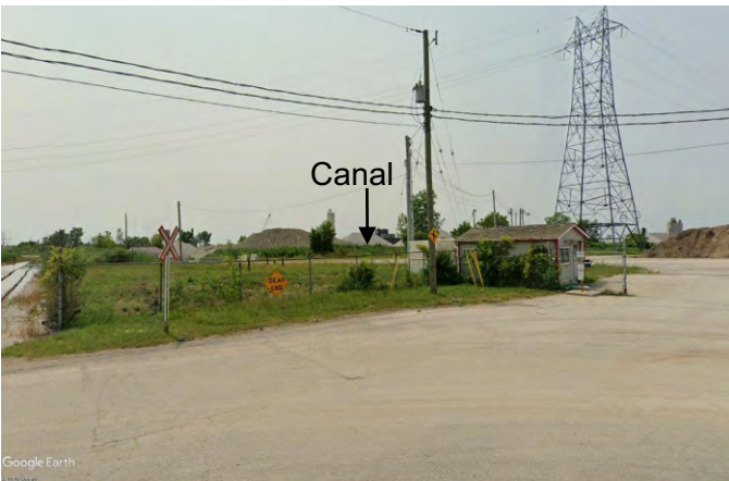
Plate 3.1-5: Prince Rd Sewer Outfall - Looking to the dead end of Russell St., with the canal and hydro tower within the Study Area in the background; facing SW (Image: Google Earth 2020, Street View, Image Date 2019).
