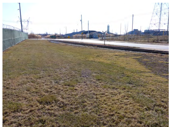
Plate 3.1-4: Prince Rd Sewer Outfall - Looking across Russell St. rail line. Note the reeds along the canal, the gate house and the berms within the fenced off portion of the Study Area: facing SW (Photo P1020120).
