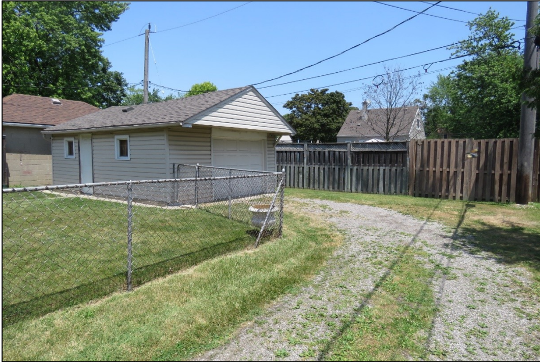
Figure 3 - Looking east towards rear detached garage at 1480 Olive Road from alley
