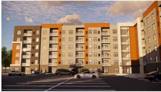
REAR - NORTH - FRONT ENTRANCE
