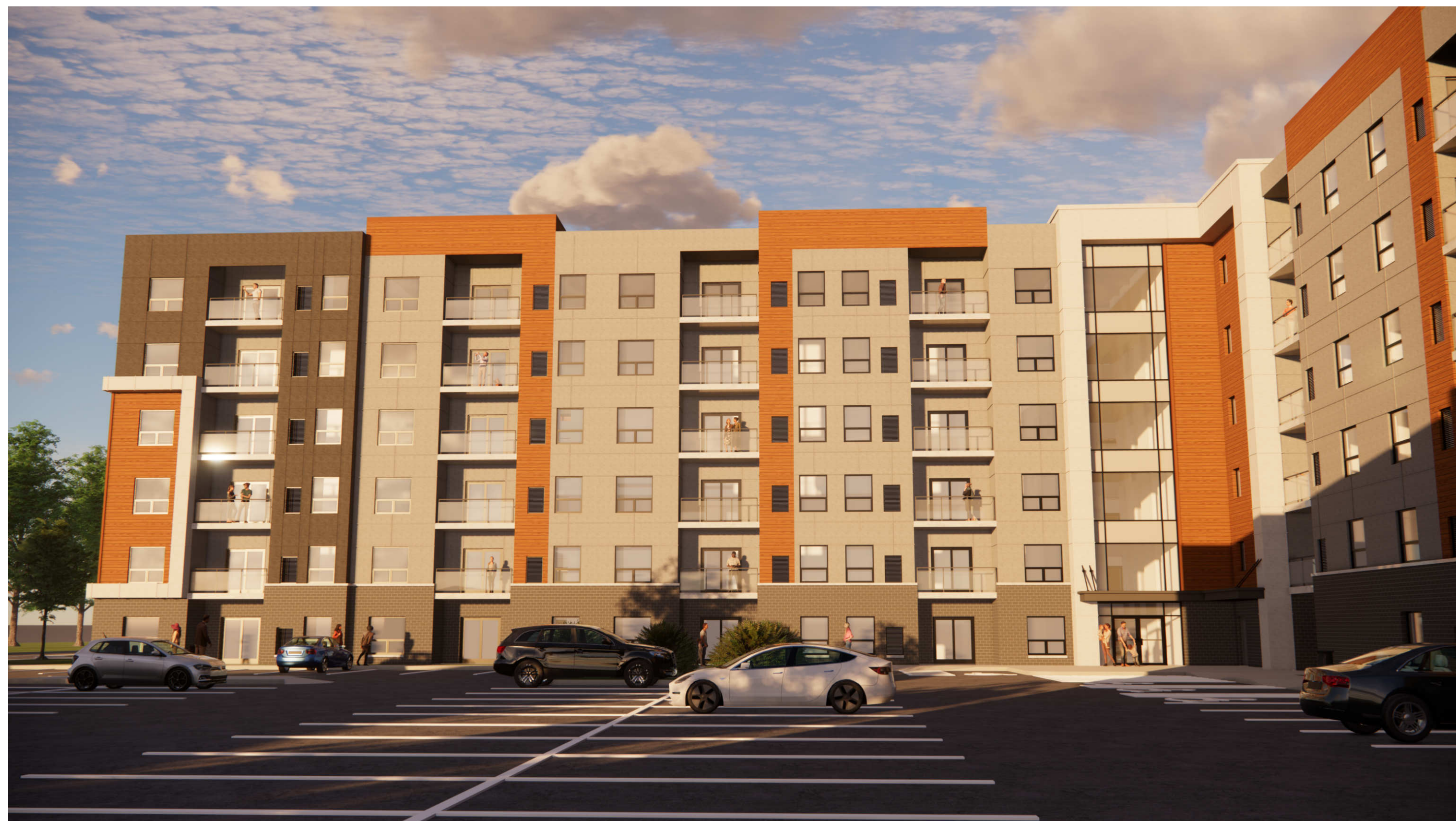
REAR - NORTH - FRONT ENTRANCE
