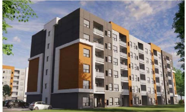
REAR - SOUTH EAST CORNER
