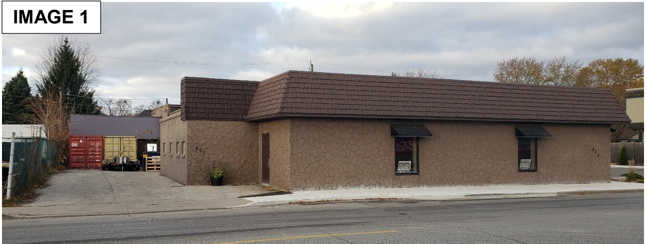
Subject Parcel – 849 Walker Road - Looking west
