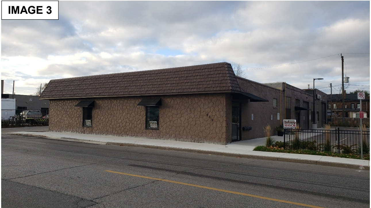
Looking southwest at Walker Road and Edna Street
