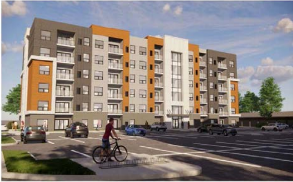
FRONT - NORTH EAST CORNER
