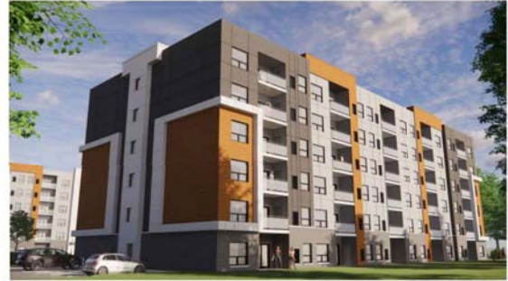
REAR - SOUTH EAST CORNER
