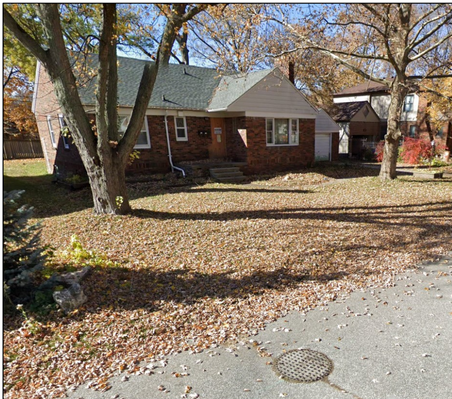
Figure 2 - Looking northwest towards 3445 Church St
