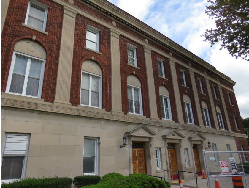
September 2023 view of the property after the limestone restoration.
