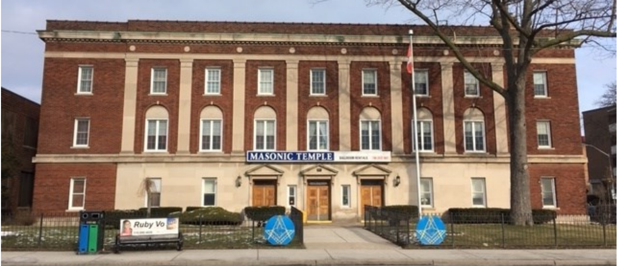
Ouellette Avenue view of the property pre-restoration.
