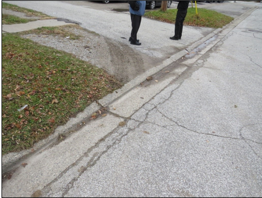
Figure 9 - Looking north towards 2321 George Ave driveway approach and Alley driveway approach
