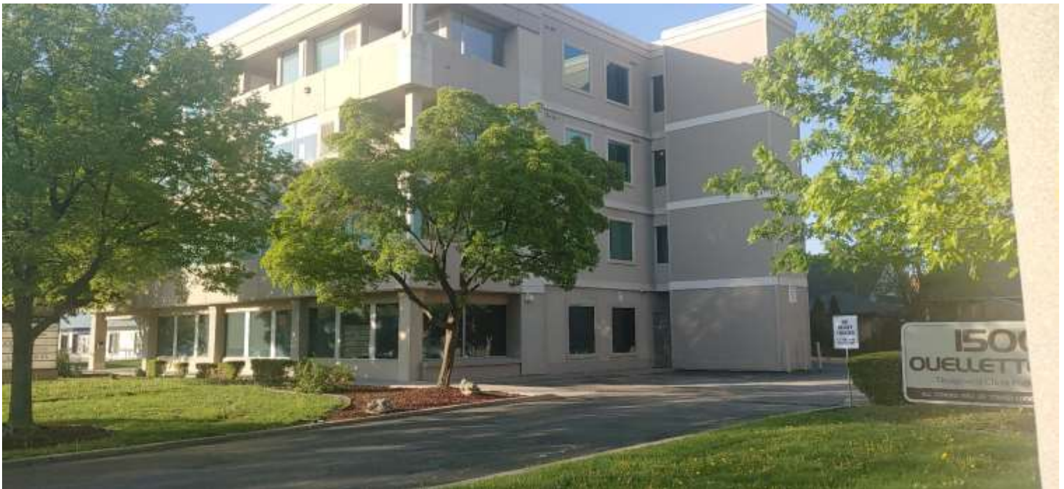
Photo 2: Ouellette Avenue View
