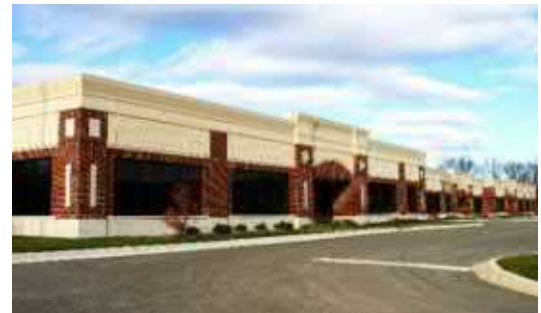
Example of elements used to indicate an entrance
