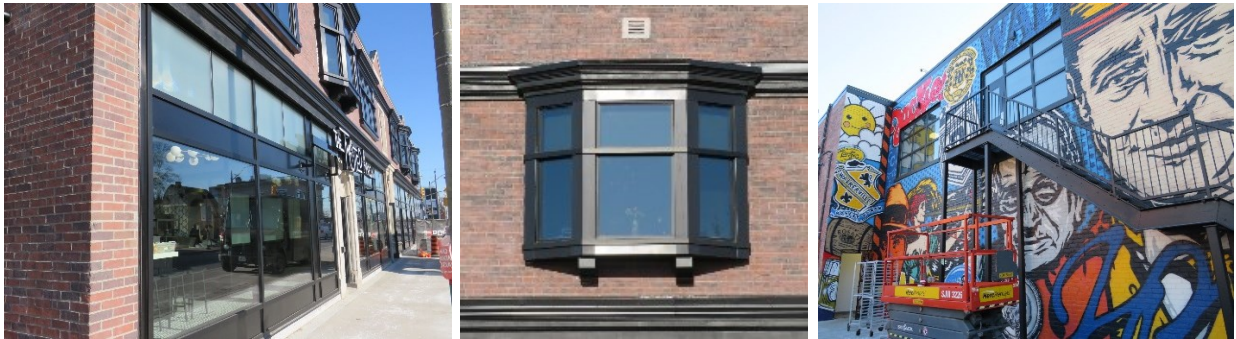
Restoration work conducted and the finished building
