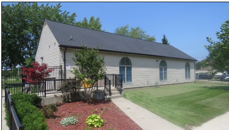
Figure 8 - Looking north towards former St. Christopher's Parish Hall from parking area
