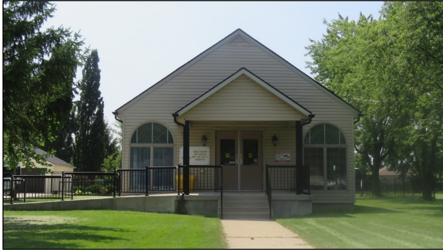
Figure 1 - Former St. Christopher's Parish Hall viewed from Woodward Boulevard
