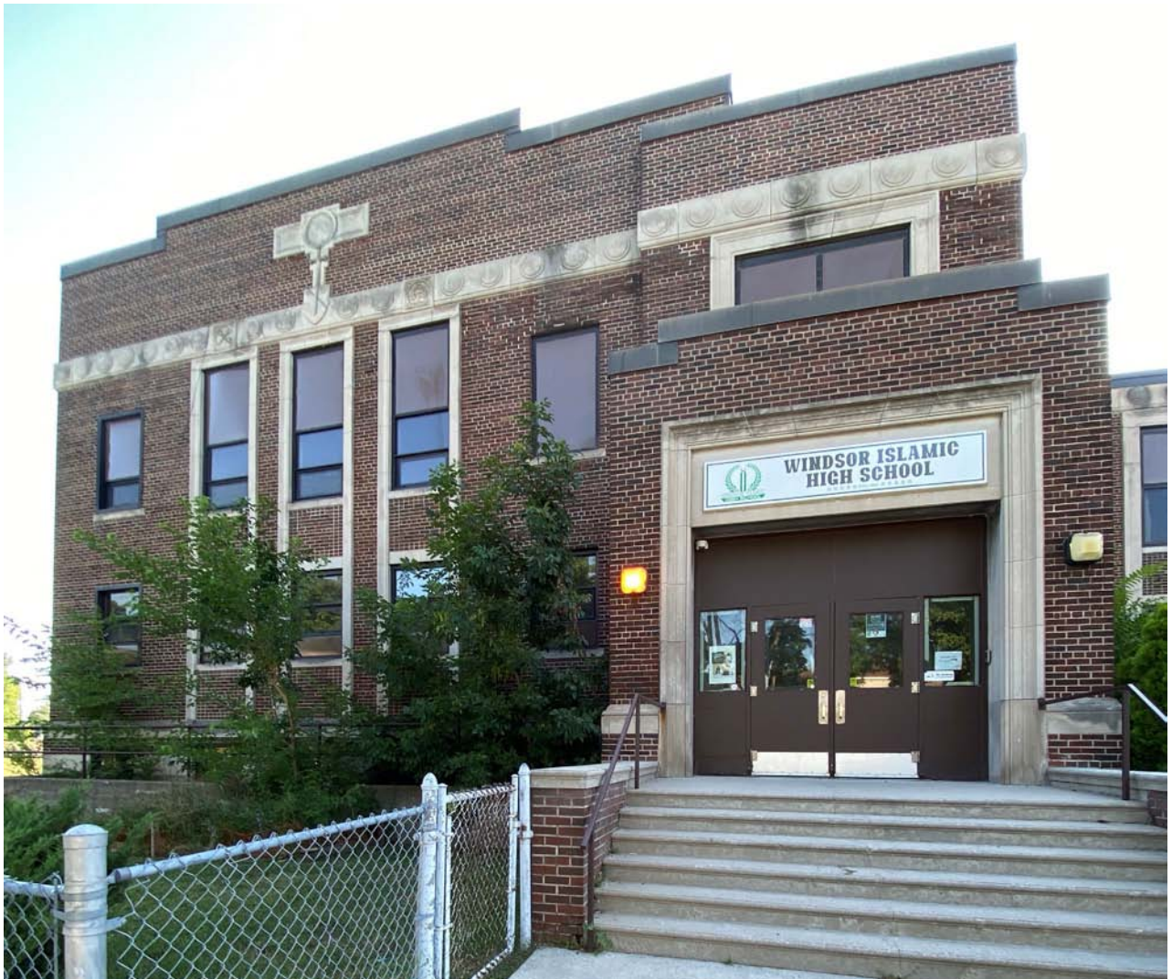
FIGURE 11: FRONT OF SCHOOL NORTH HALF
