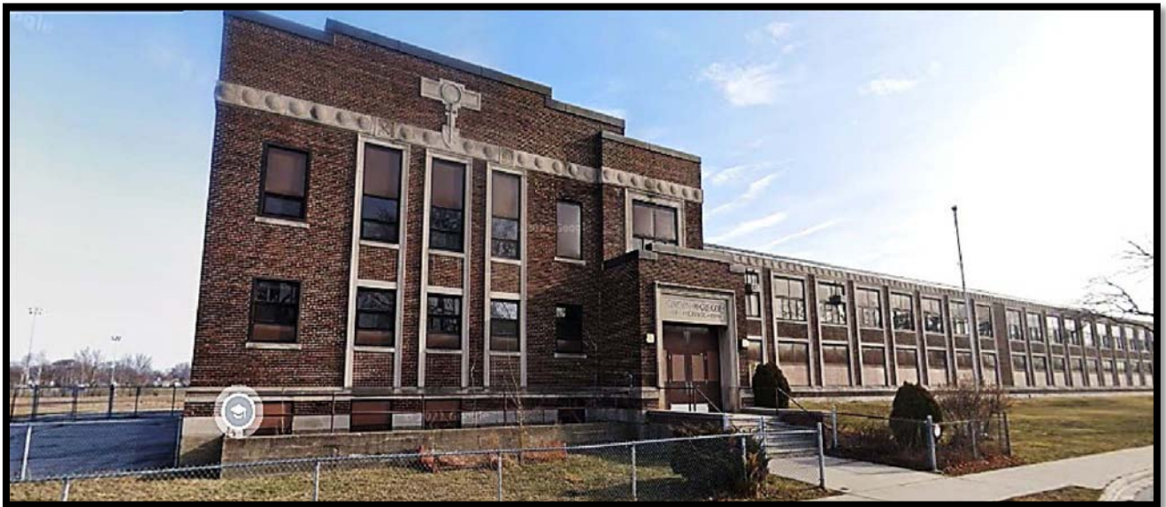
FIGURE 6 – FORMER GORDON MCGREGOR ELEMENTARY SCHOOL, 2021
