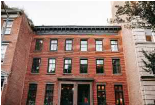
Example of architectural articulations and window fenestrations
