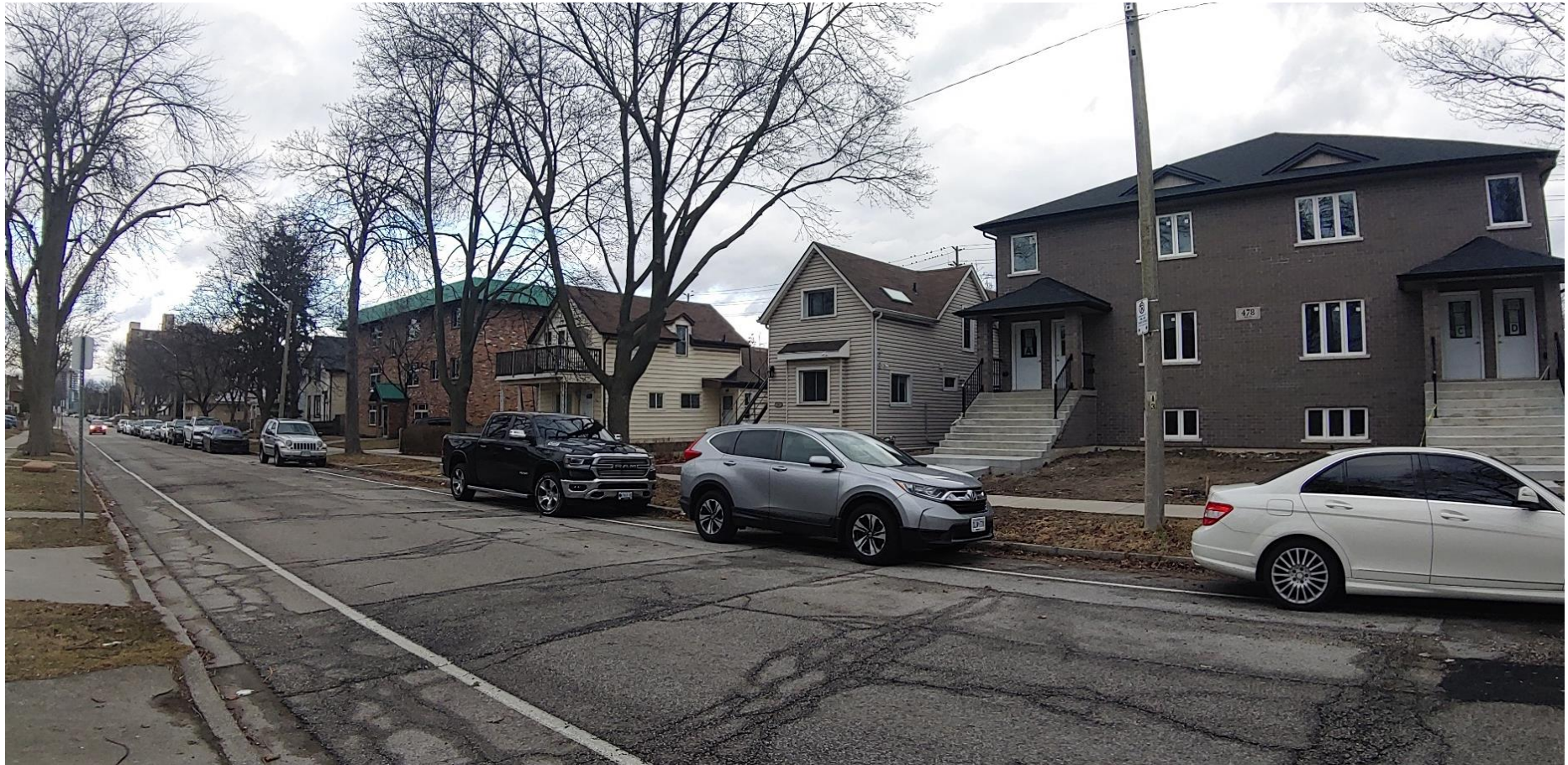
View of existing buildings on the E/S of Janette Ave. N/S of subject 4-plex at 478 Janette Ave.
