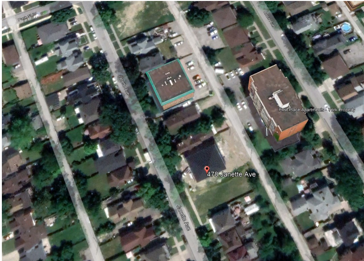
New Building (under construction) at 478 Janette Avenue, on Google Earth Photo, Jun 2022
