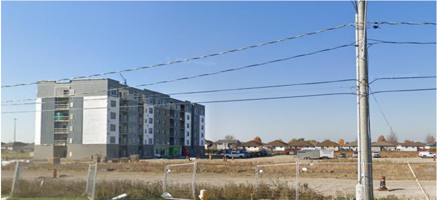
View of East and North Walls of Building 2
