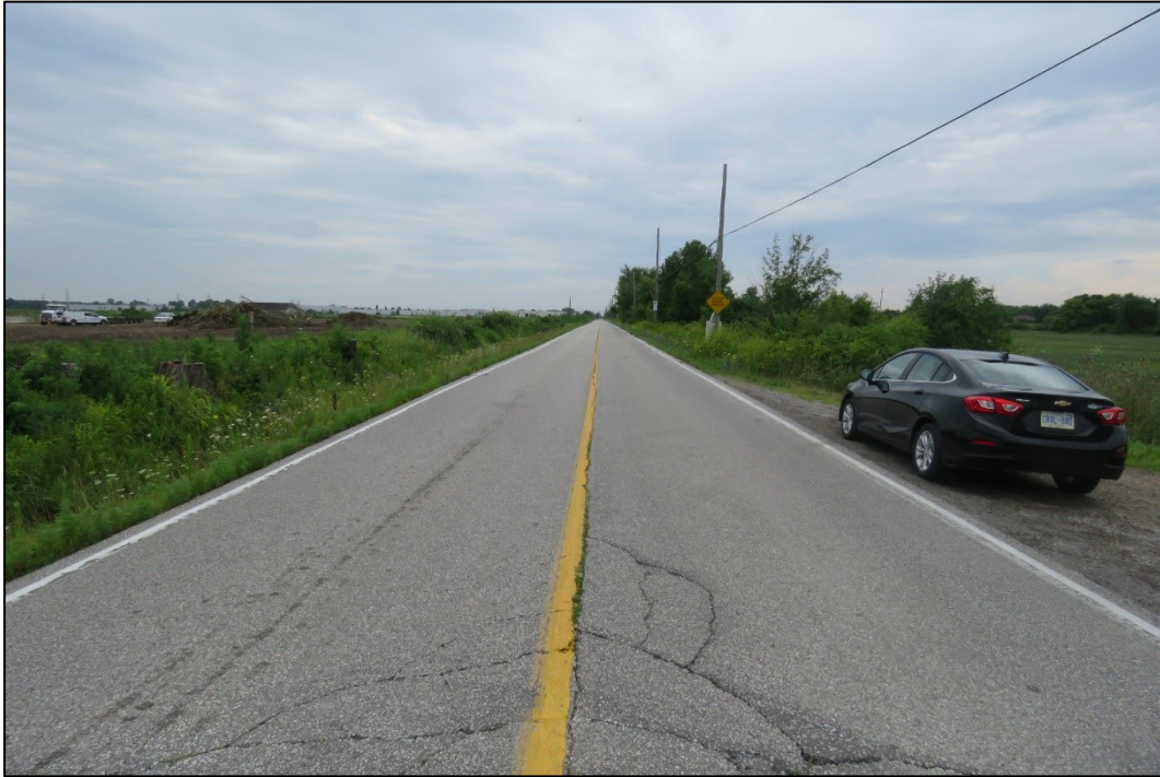
Figure 5 - E. C. Row Avenue East looking west from Banwell Road 1
