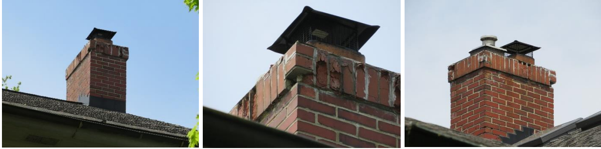
Close-up views of the north chimney
