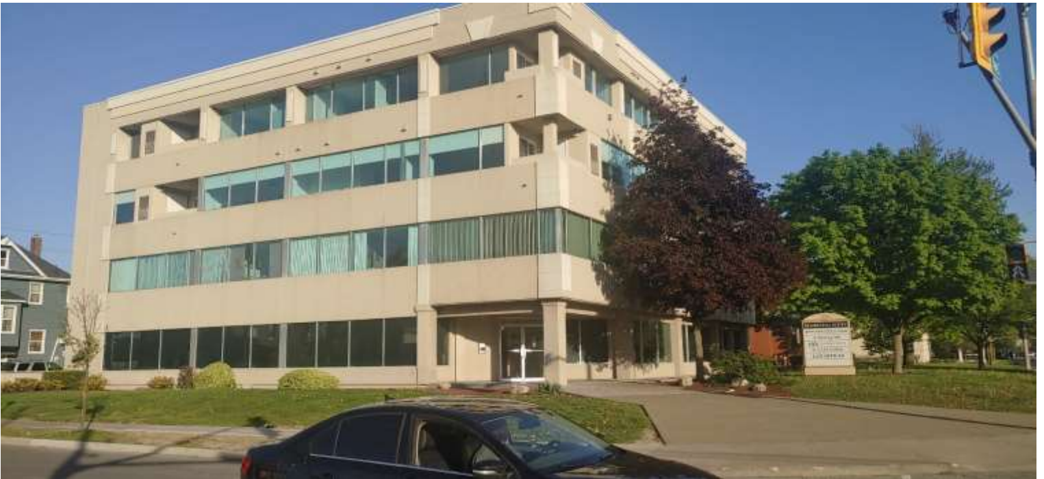
Photo 4: Close View of main pedestrian entrance off Ouellette & Shepherd
