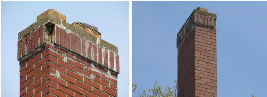
Close-up views of the central chimney
