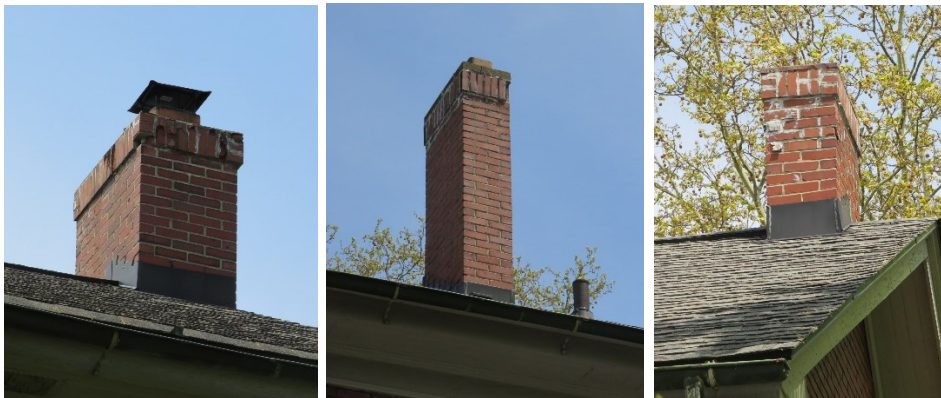
Photos of the three chimneys (taken May 8, 2023)
