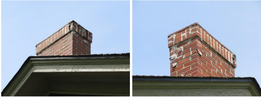
Close-up views of the south chimney
