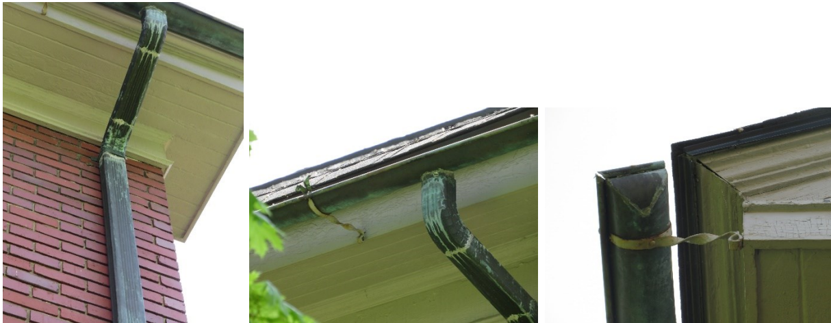
Photos of the gutter system (taken May 8, 2023)
