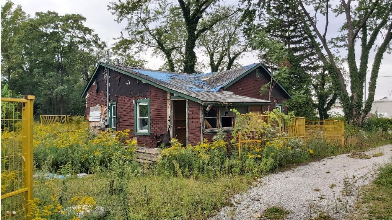
Subject Site, Abandoned house
