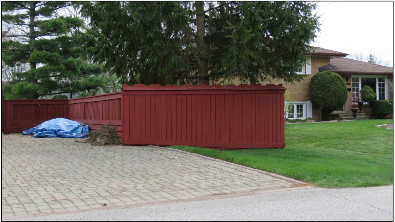
Figure 7 - Looking south towards north/south alley from Joinville Avenue (5097 Joinville Avenue on right)
