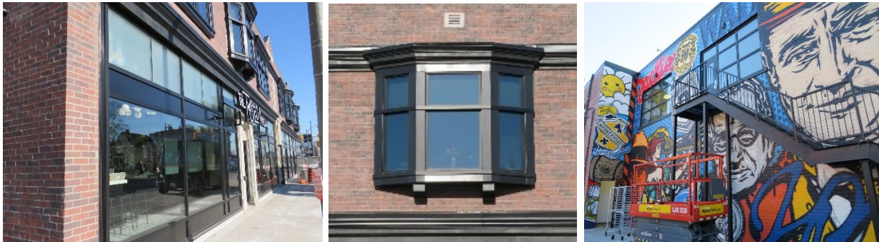
Restoration work conducted and the finished building
