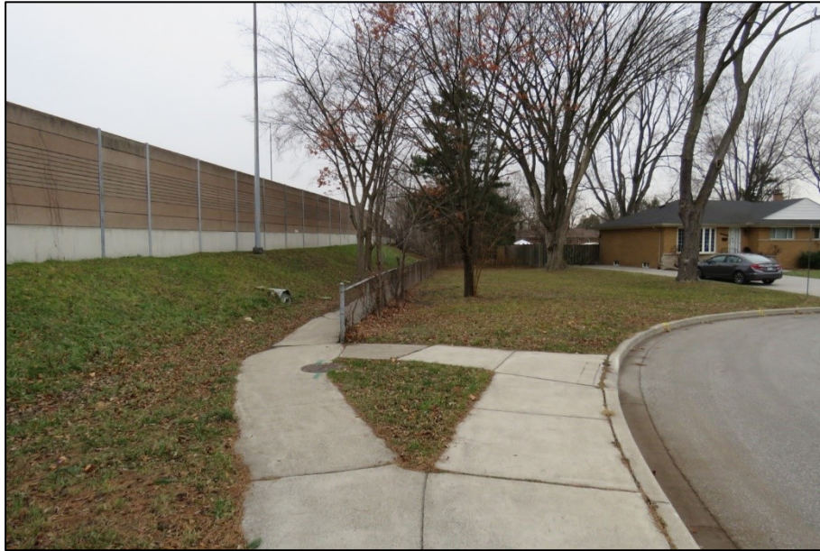
Figure 1 - Looking west towards east/west alley from Academy Drive (2589 Academy Drive on right)
