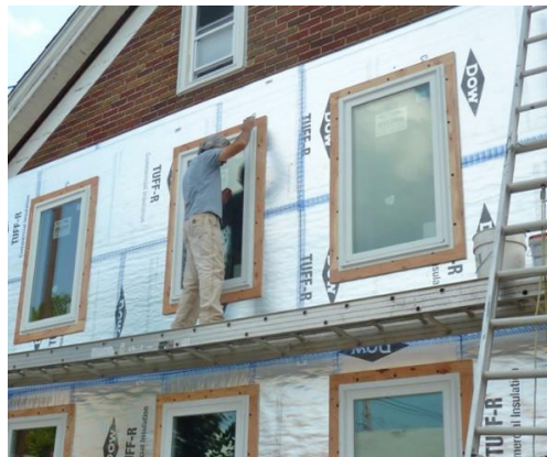
Figure 13: Example of exterior upgrades to existing home
