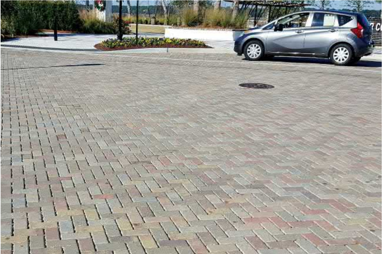
Example of sustainable design, which incorporates permeable pavement to help with stormwater management 1
