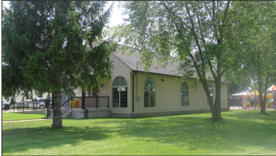
Figure 3 - Looking southwest towards former St. Christopher's Parish Hall from Woodward Boulevard
