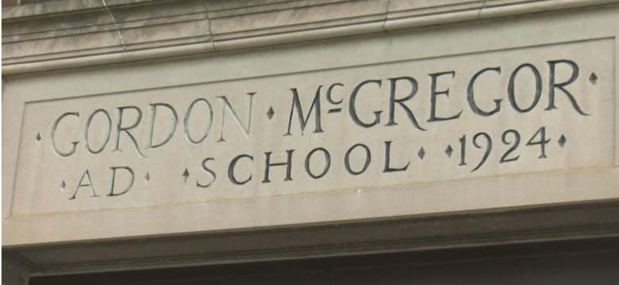
FIGURE 35: FRONT FAÇADE KEYSTONE
