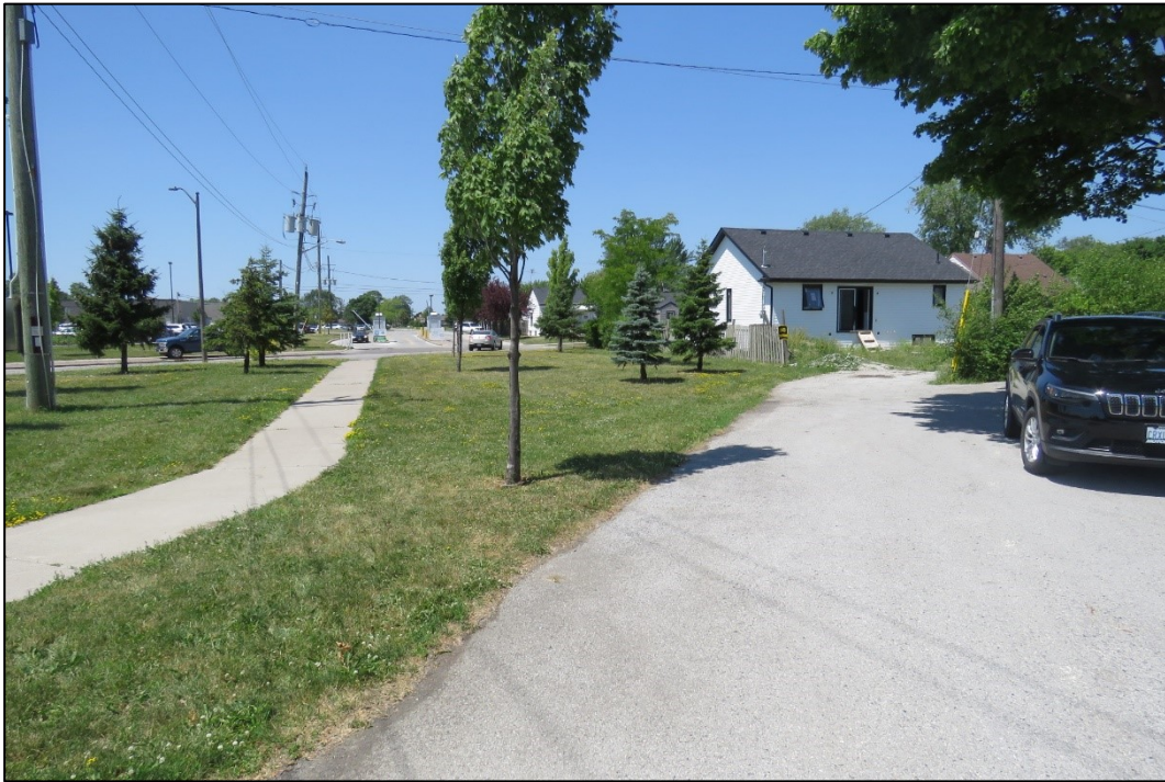
Figure 3 - Looking north towards Lillian Street right-of-way from Memorial Drive
