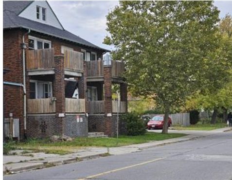
Front view of 561 Parent Avenue, looking west from Parent Avenue
