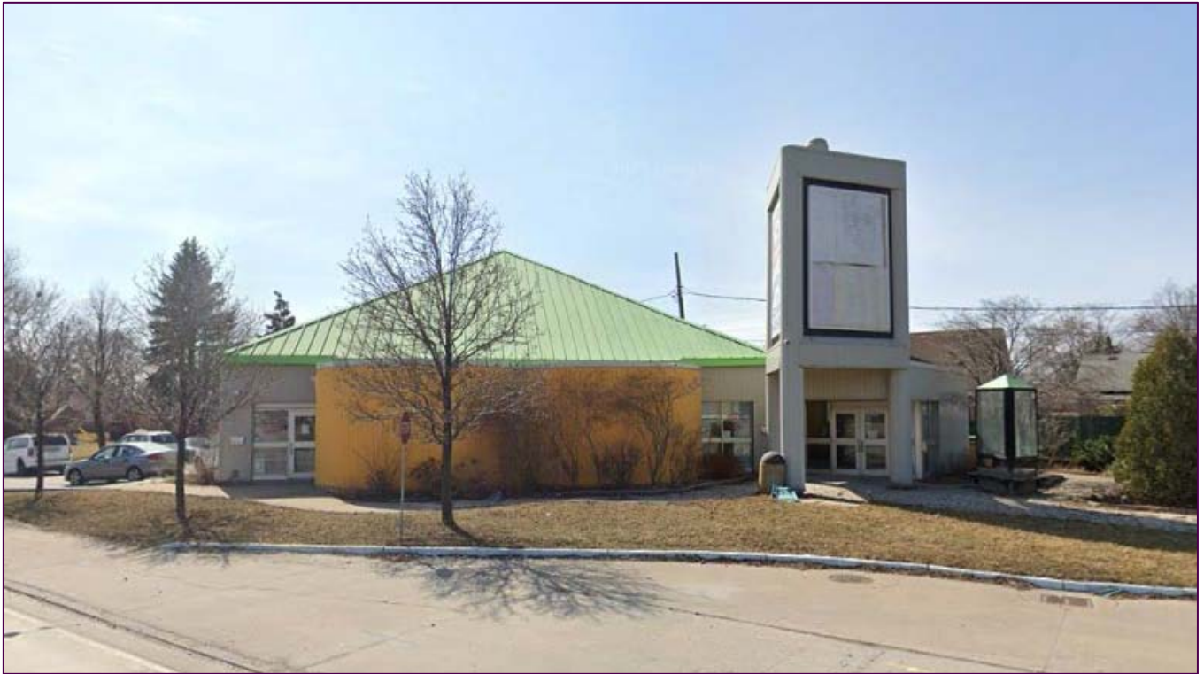
FIGURE 4 - EXISTING BUILDING (FORMER TOURIST BUREAU)
