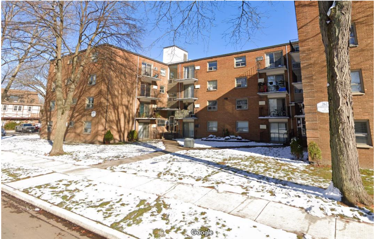
Figure 17 - Example of Accessible Outdoor Amenity Space (260 & 262 Randolph Place)
