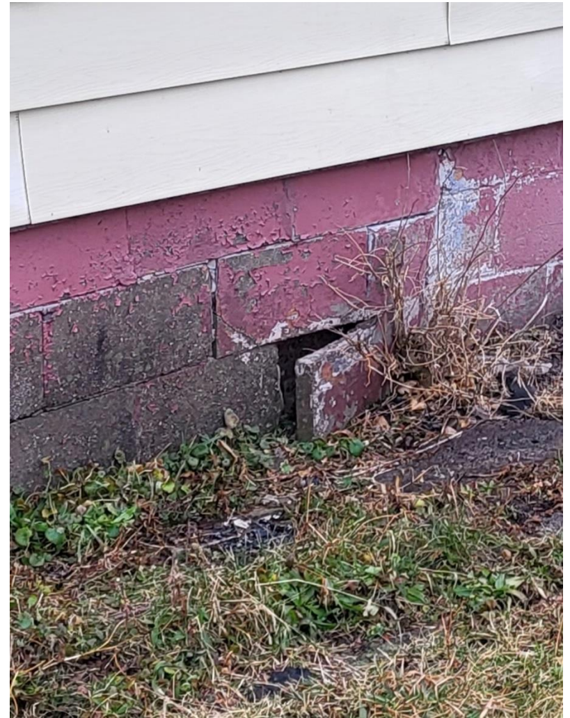
8. Foundation wall close up at side of building (West elevation).
