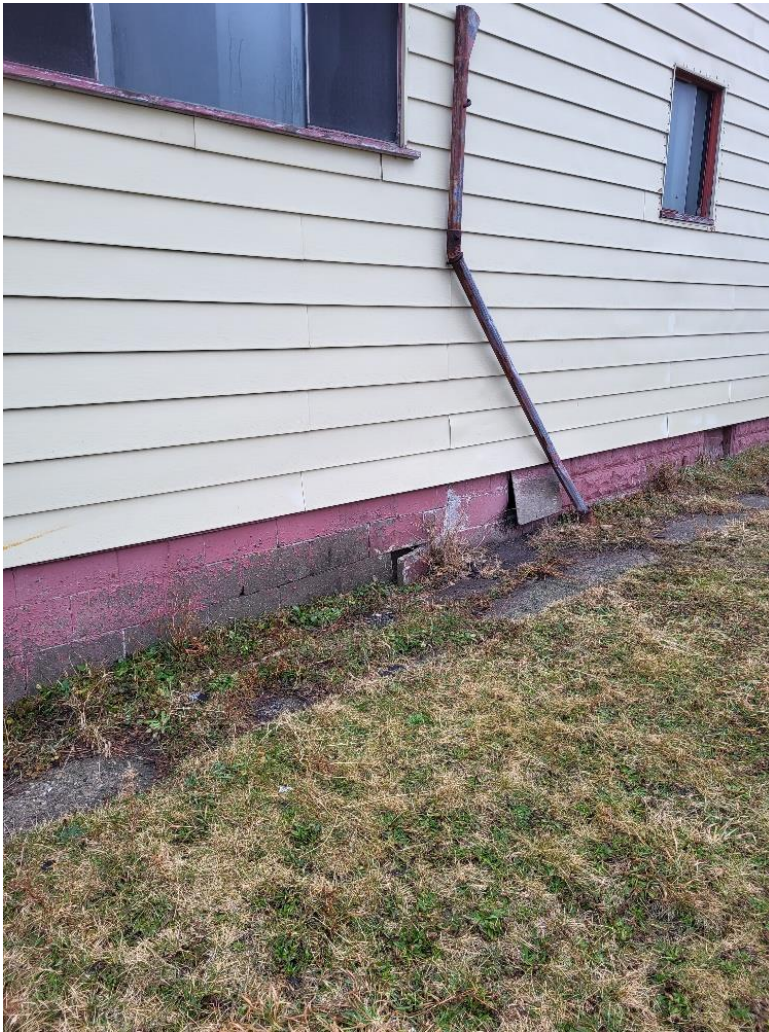
7. Side of building (West elevation).
