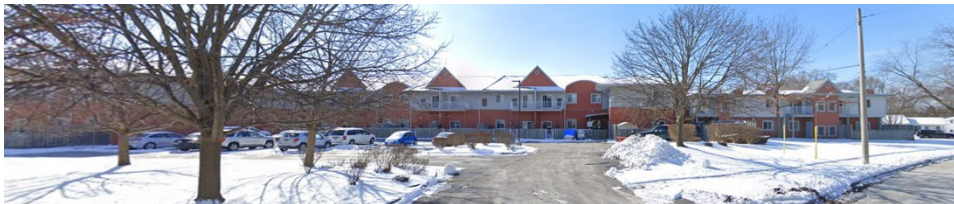
Former Ivor Chandler School (Source: Google Streetview)
