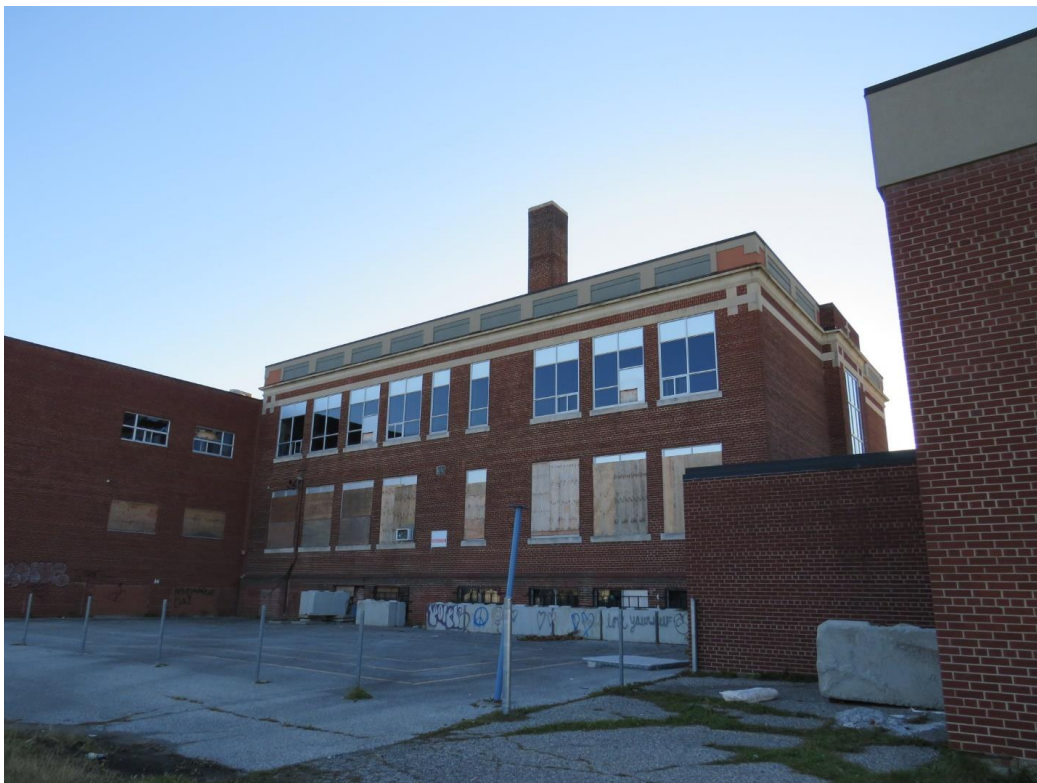
Rear of original construction
