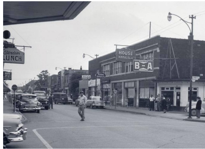
Example of projecting wall signs on Buildings at the intersection of Whelpton Street and Drouillard Road in the 1950s.
