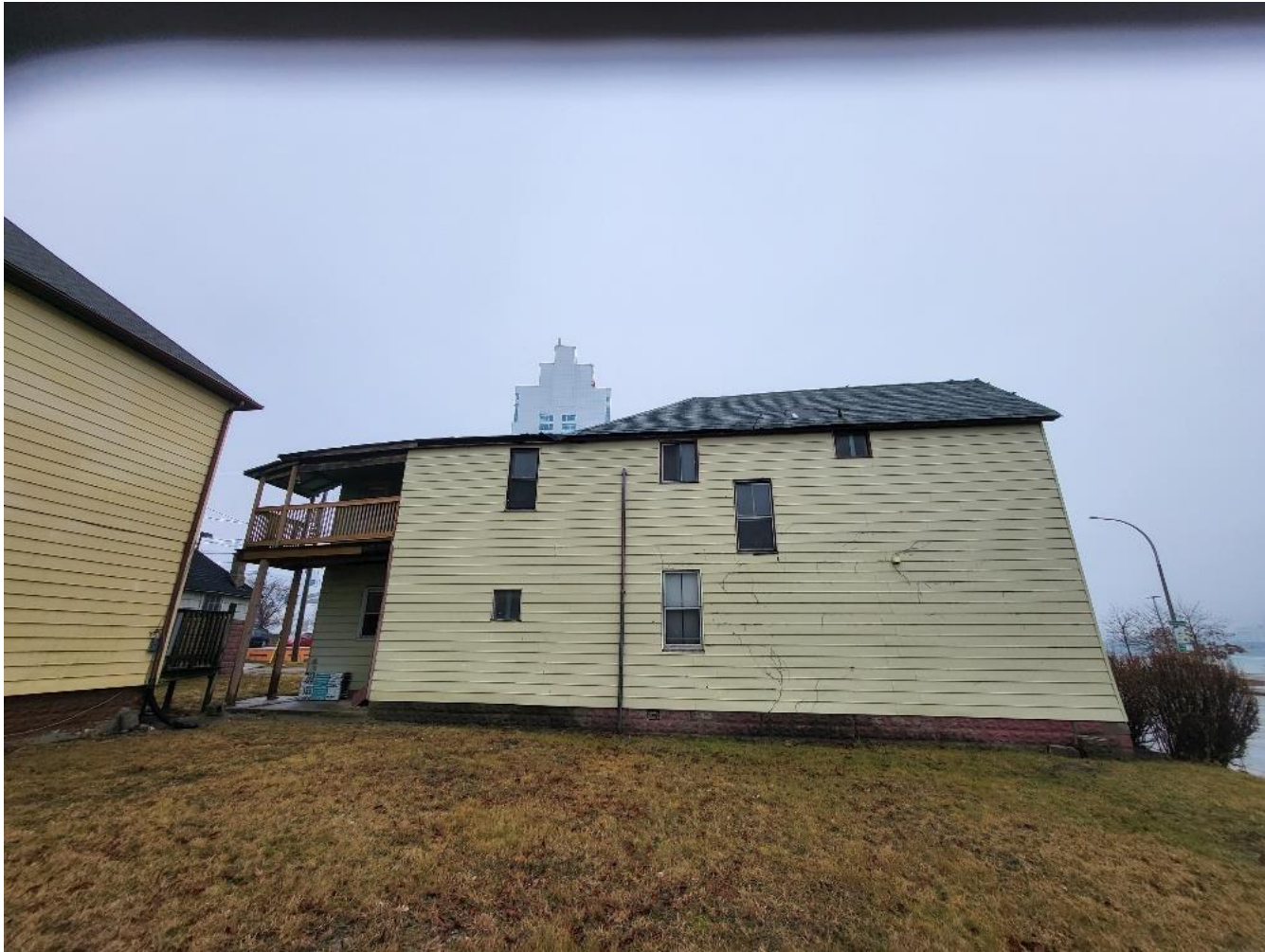
4. Side of building (East elevation).
