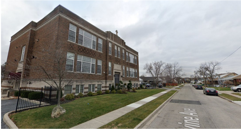
Former Ste. Genevieve School (Source: Google Streetview)
