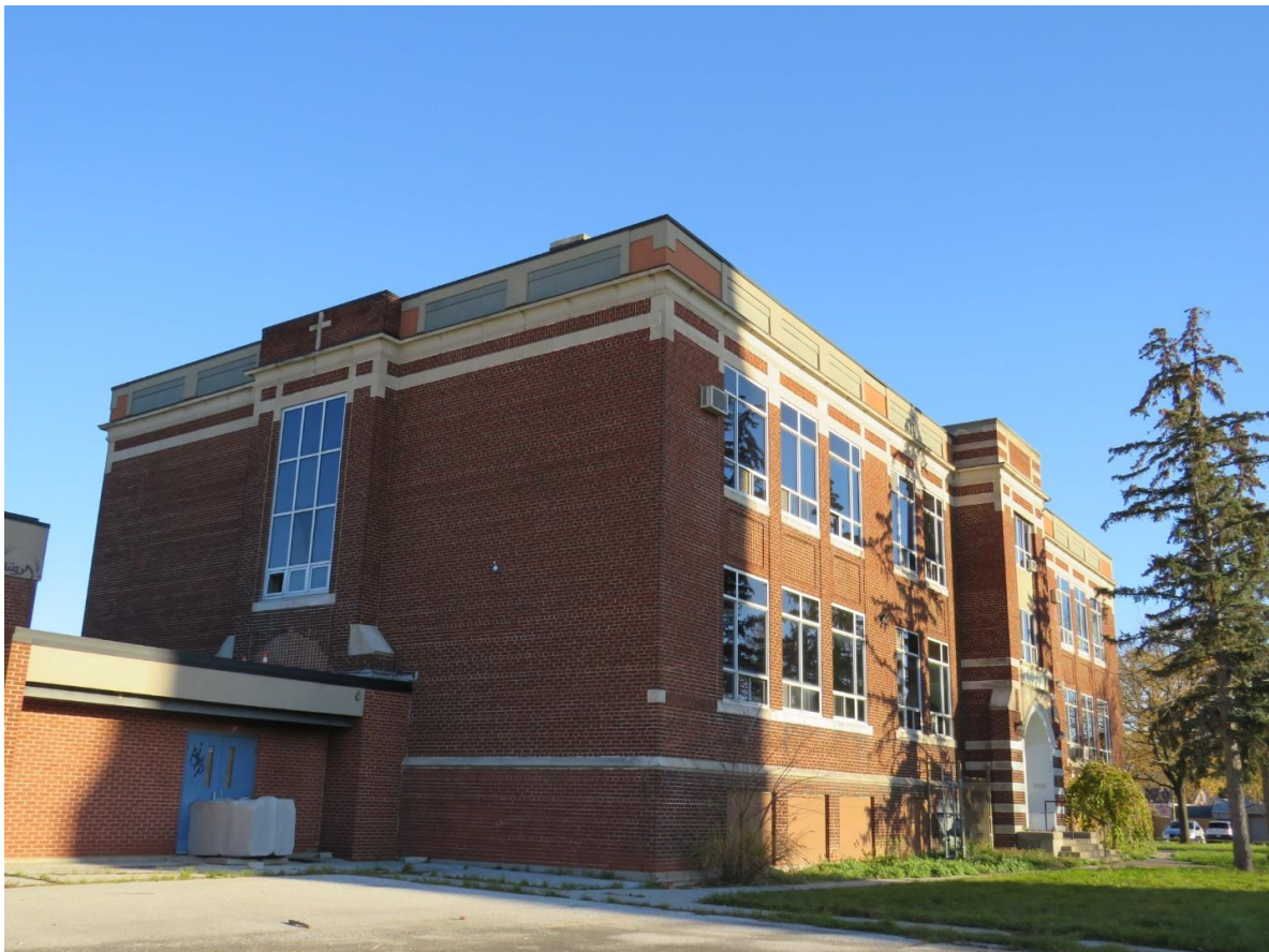
Northwest corner of property showing 1965 Gymnasium addition
