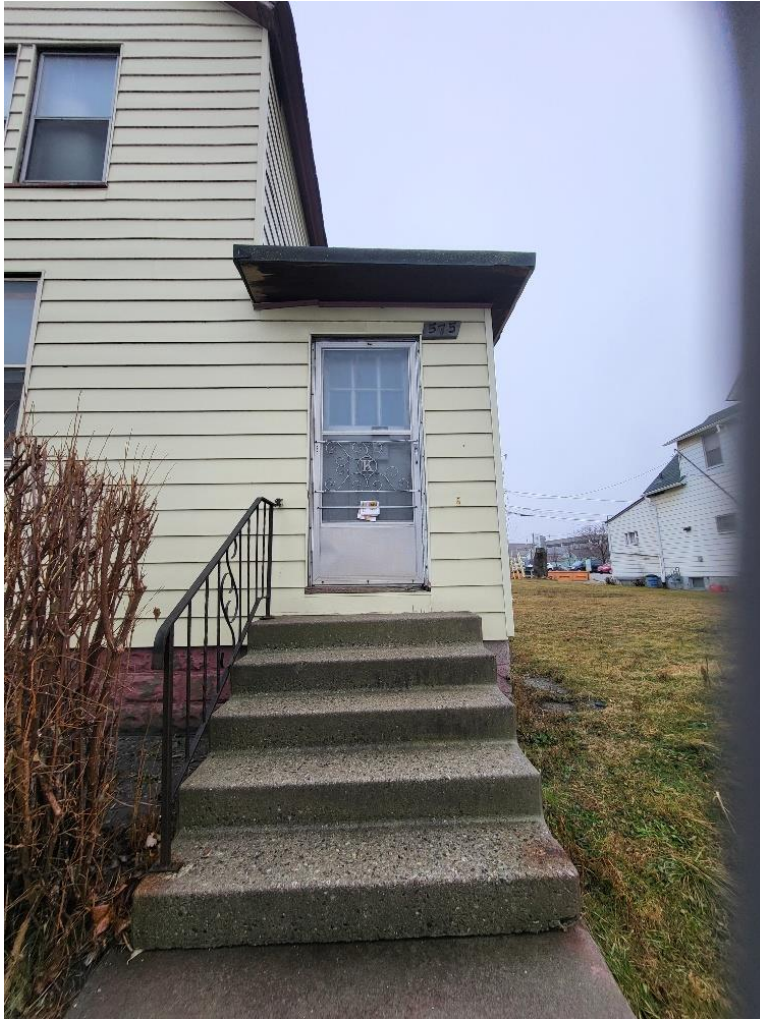
2. Front of building (North elevation).
