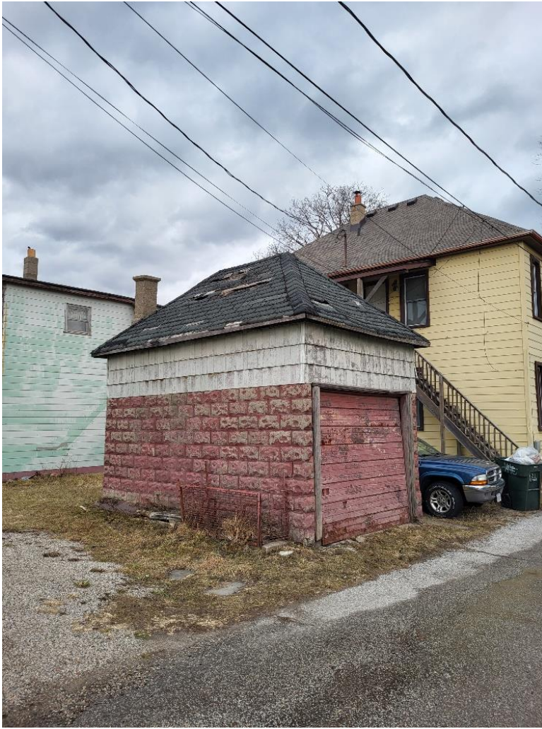
1. Rear accessory structure.
