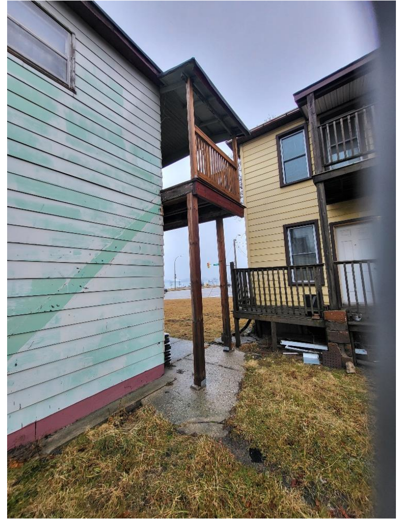
3. Rear of building (South elevation).
