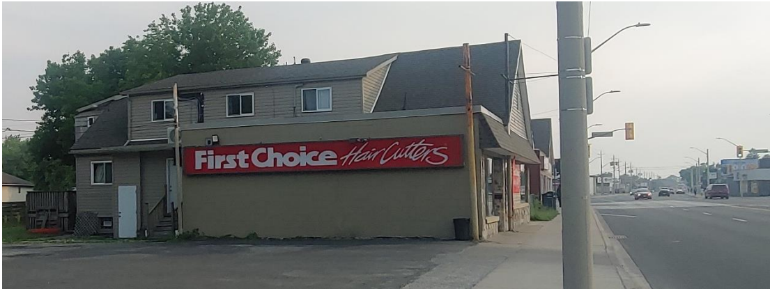
Photo No. 5 – View of the abutting building (First Choice Haircutters) on the west side of the subject land
