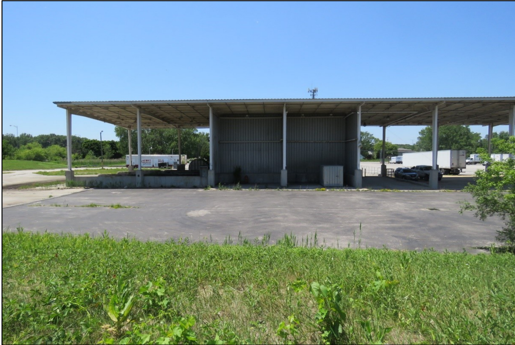
Figure 3 - Outdoor storage yard at Penske Truck Rental
