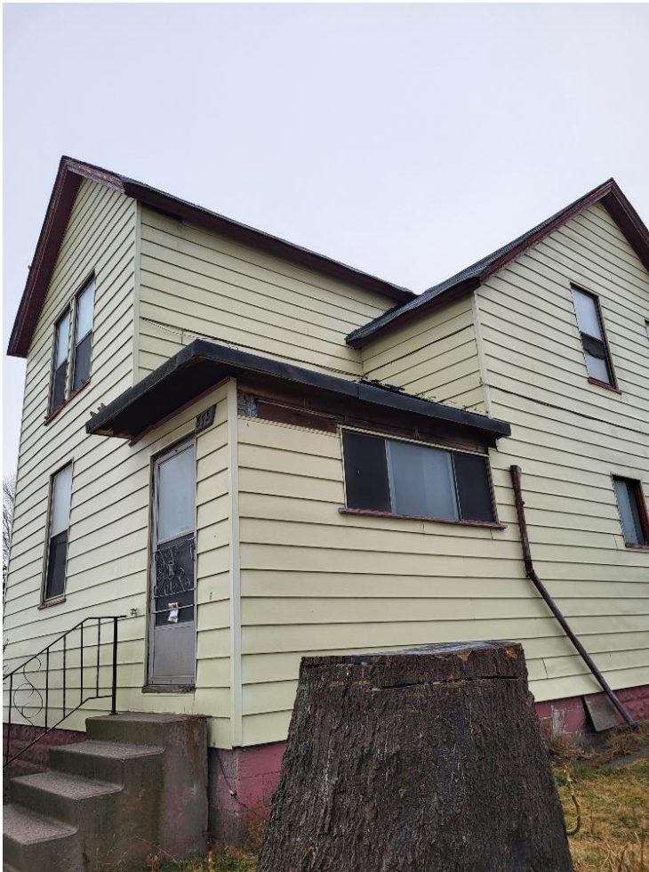
5. Side of building (West elevation).
