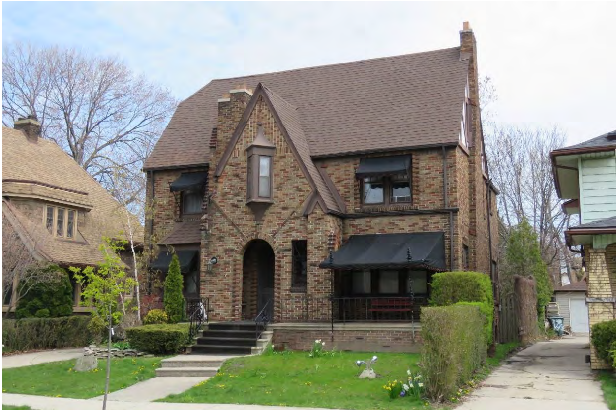
Front elevation of 436 Askin Ave.
