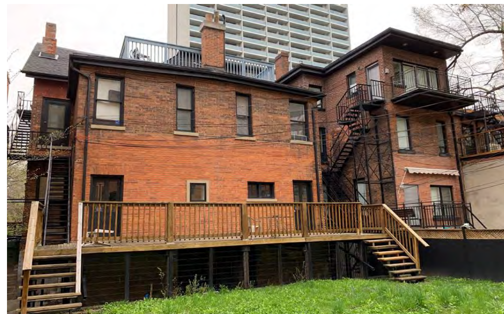
Rear (south) elevation of 29-31 Prince Arthur Avenue (ERA Architects, 2022)
